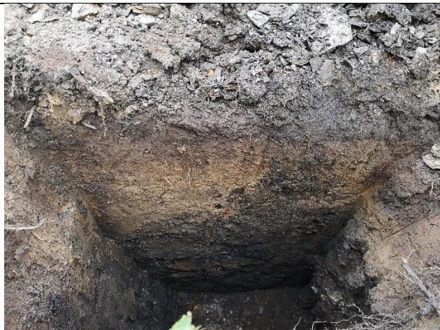
Trial Pit 6: Internal view of excavation
