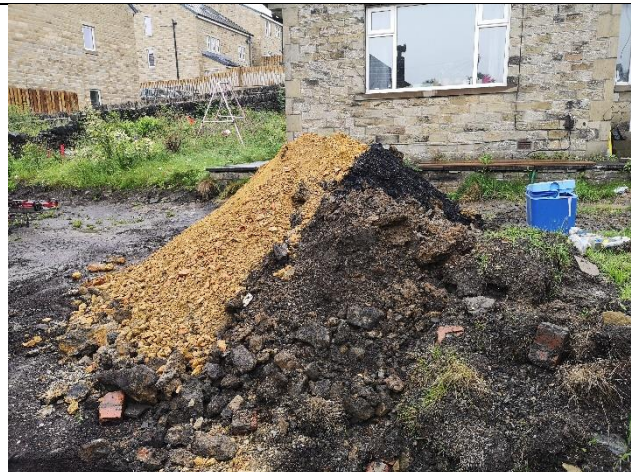
Trial Pit 13: Overview of excavated soils
