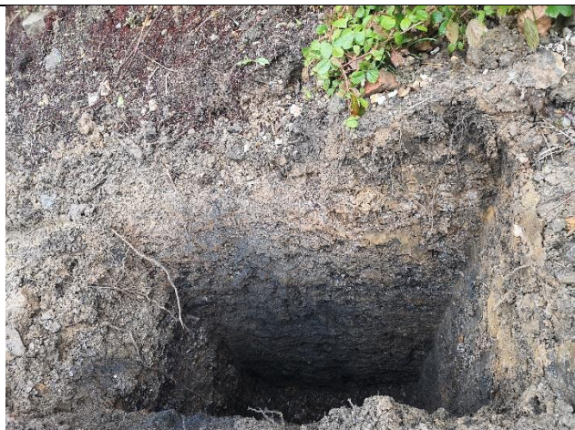
Trial Pit 8: Internal view of excavation
