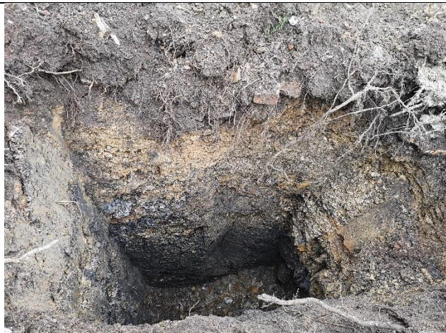
Trial Pit 8: Internal view of excavation
