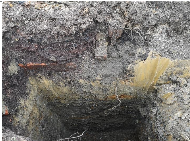
Trial Pit 8: Internal view of excavation
