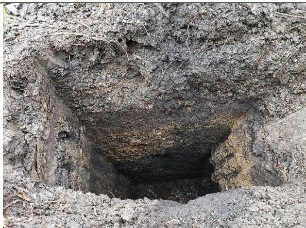
Trial Pit 4: Internal view of excavation
