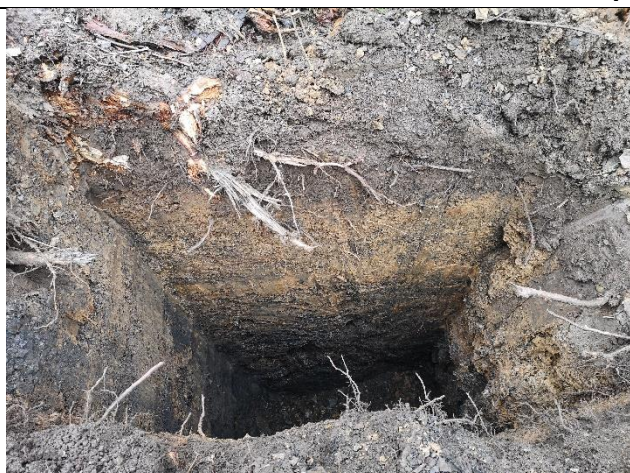
Trial Pit 3: Internal view of excavation
