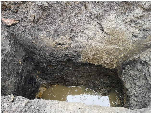
Trial Pit 15: Internal view of excavation
