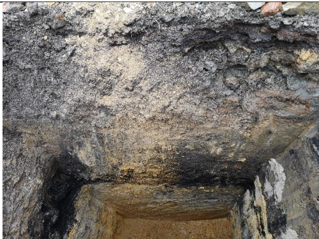
Trial Pit 13: Internal view of excavation
