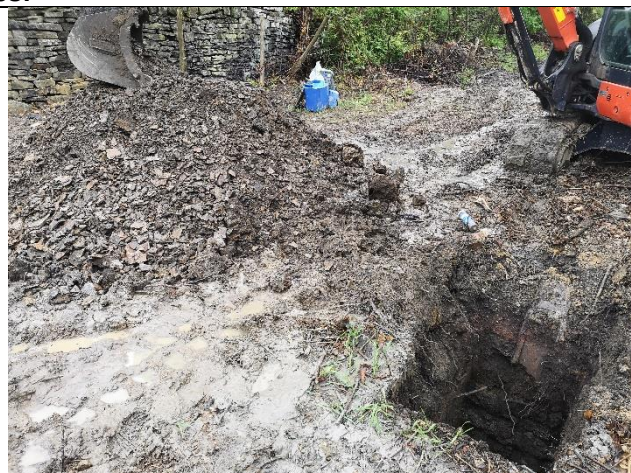
Trial Pit 7: Overview of excavated soils
