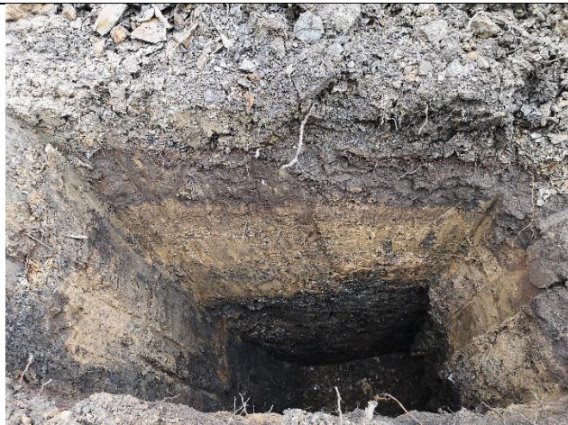
Trial Pit 5: Internal view of excavation
