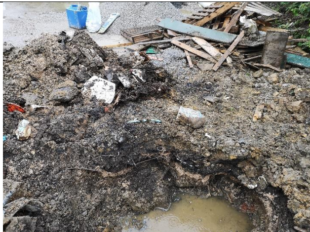
Trial Pit 12: Internal view of excavation
