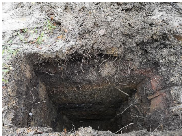
Trial Pit 7: Internal view of excavation
