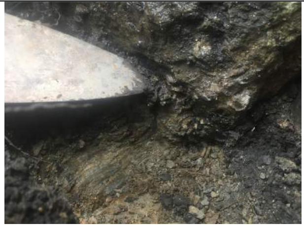
Plate 8 – The contact between the concrete foundation and underlying sandstone bedrock.
