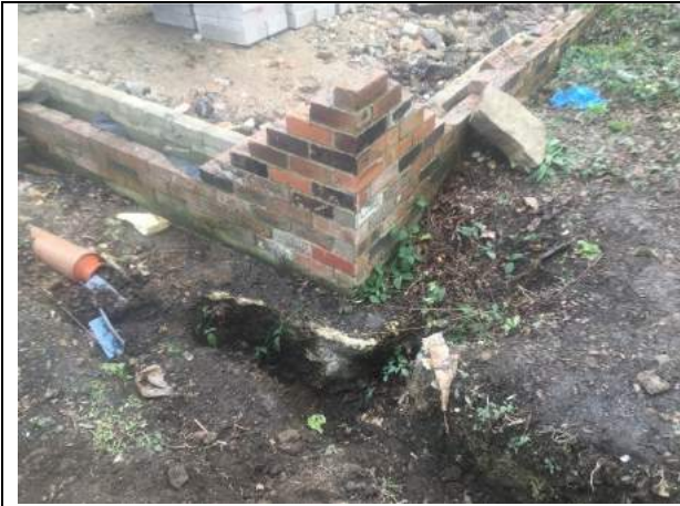
Plate 7 – The NW corner of the existing extension foundations.
