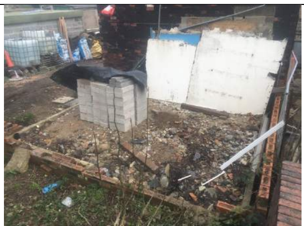
Plate 4 – The existing extension, the centre of the foundations infilled with Made Ground.
