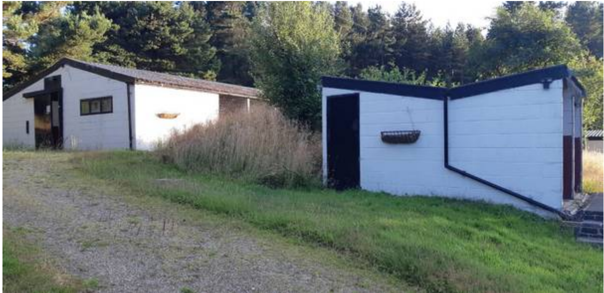
Figure 4: Existing buildings 1 and 3
