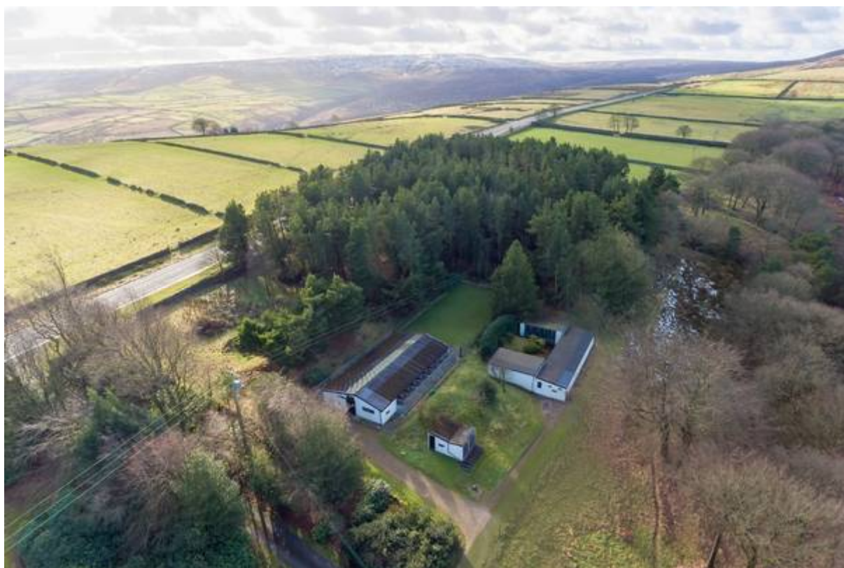
Figure 3: Close-up aerial view of site
