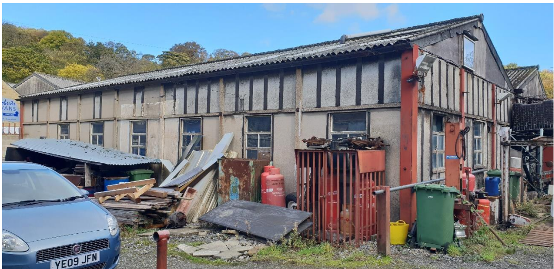
Existing West Elevation (Side) of Building
