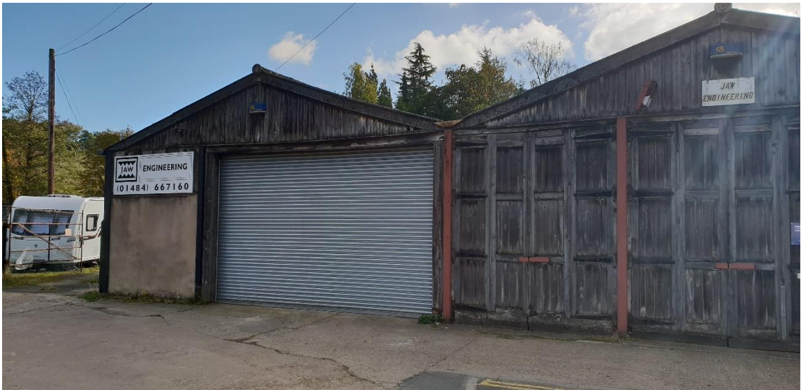
Existing North Elevation (Front) of Building
