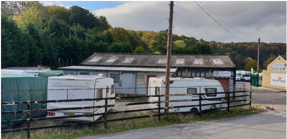
Proposed site as viewed from Existing access
