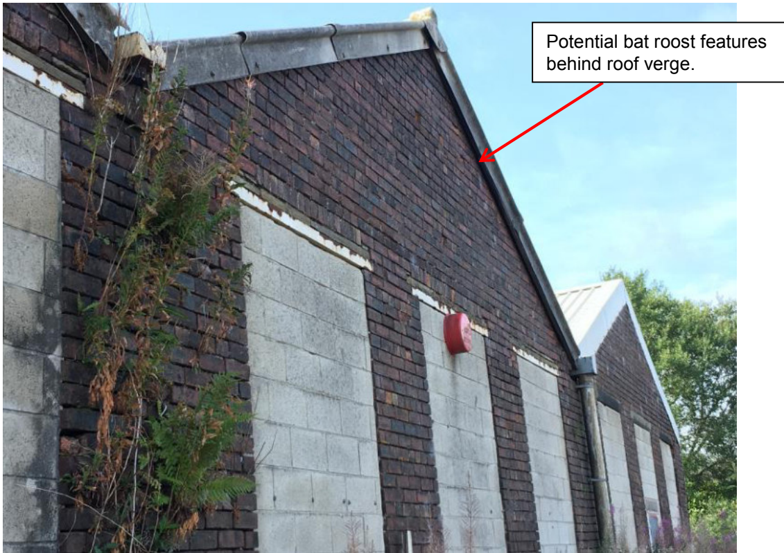
Photo 7. Northern elevation of building on the site
