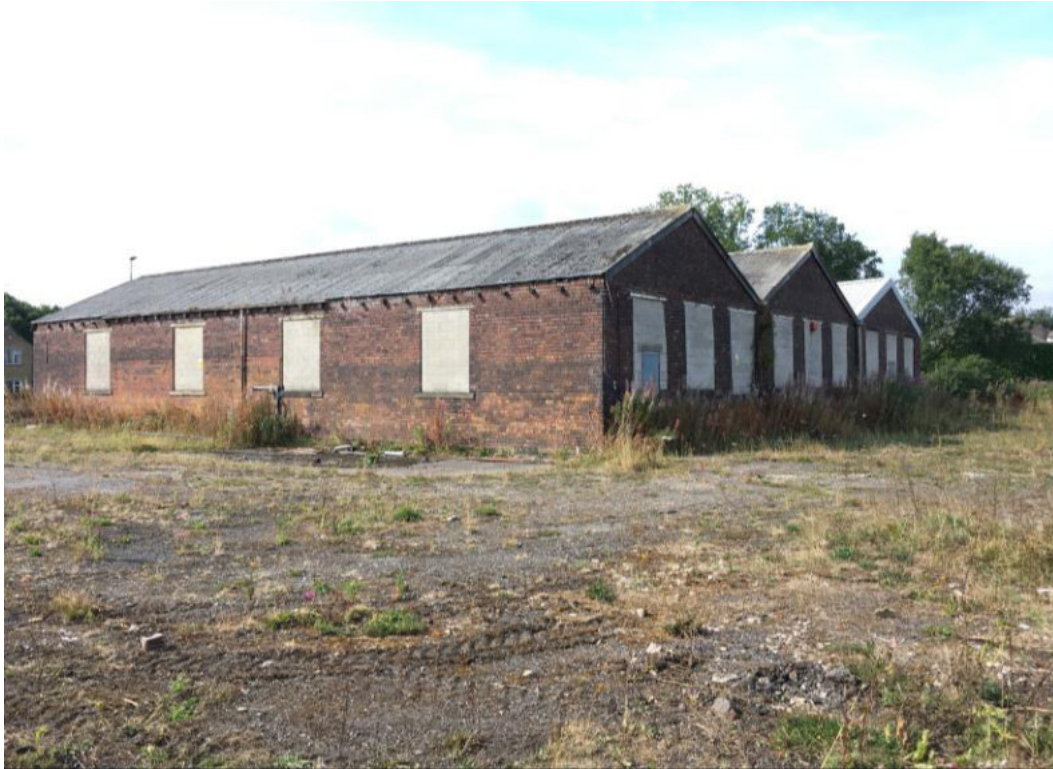
Photo 1. Looking south-west towards the building on the site
