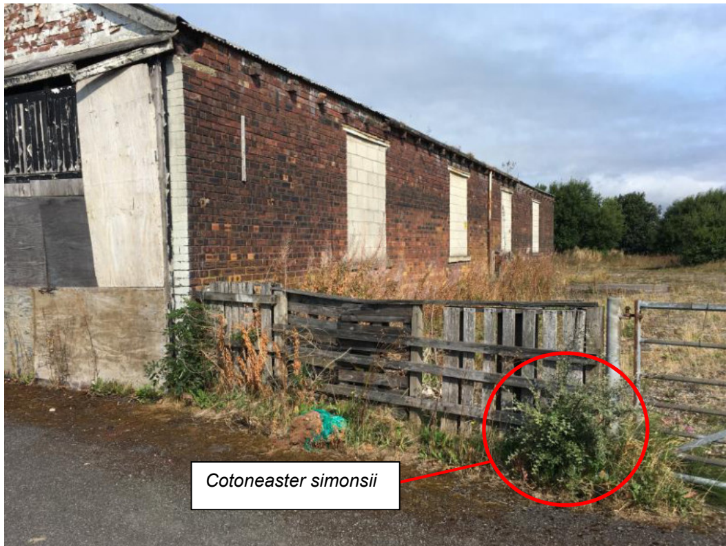
Photo 2. Looking north-west along eastern elevation of the building on the site
