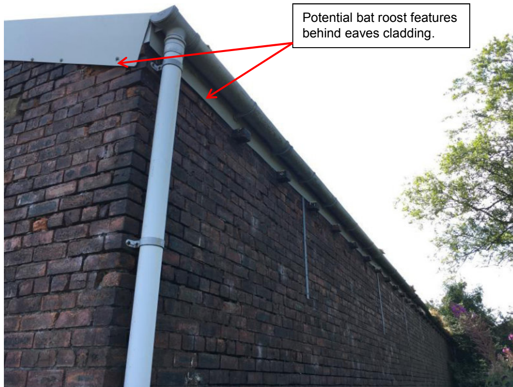
Photo 6. Western elevation of building on the site
