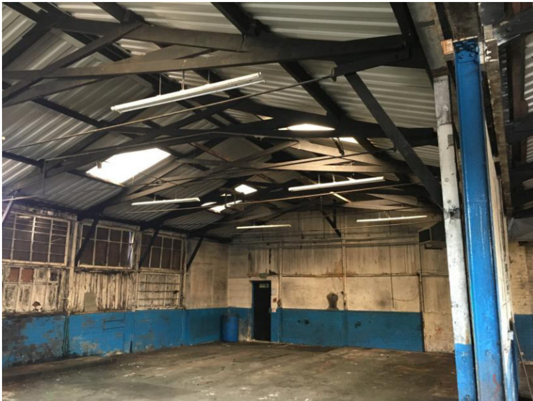
Photo 12. Interior of building (western part)
