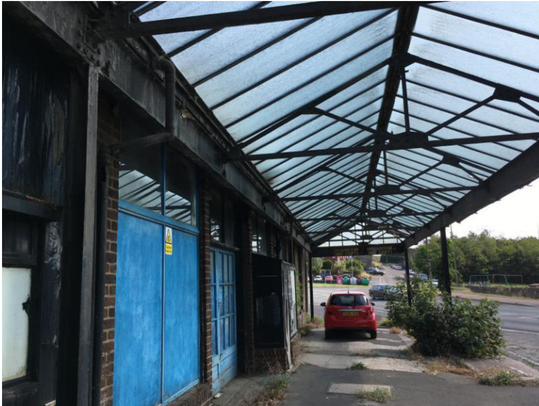
Photo 11. Glass canopy on south elevation of building
