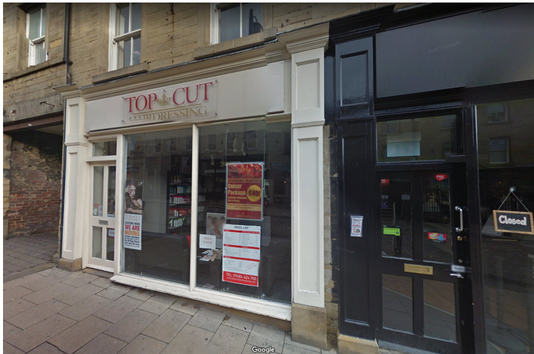
Existing Shop 49 King Street, Huddersfield
