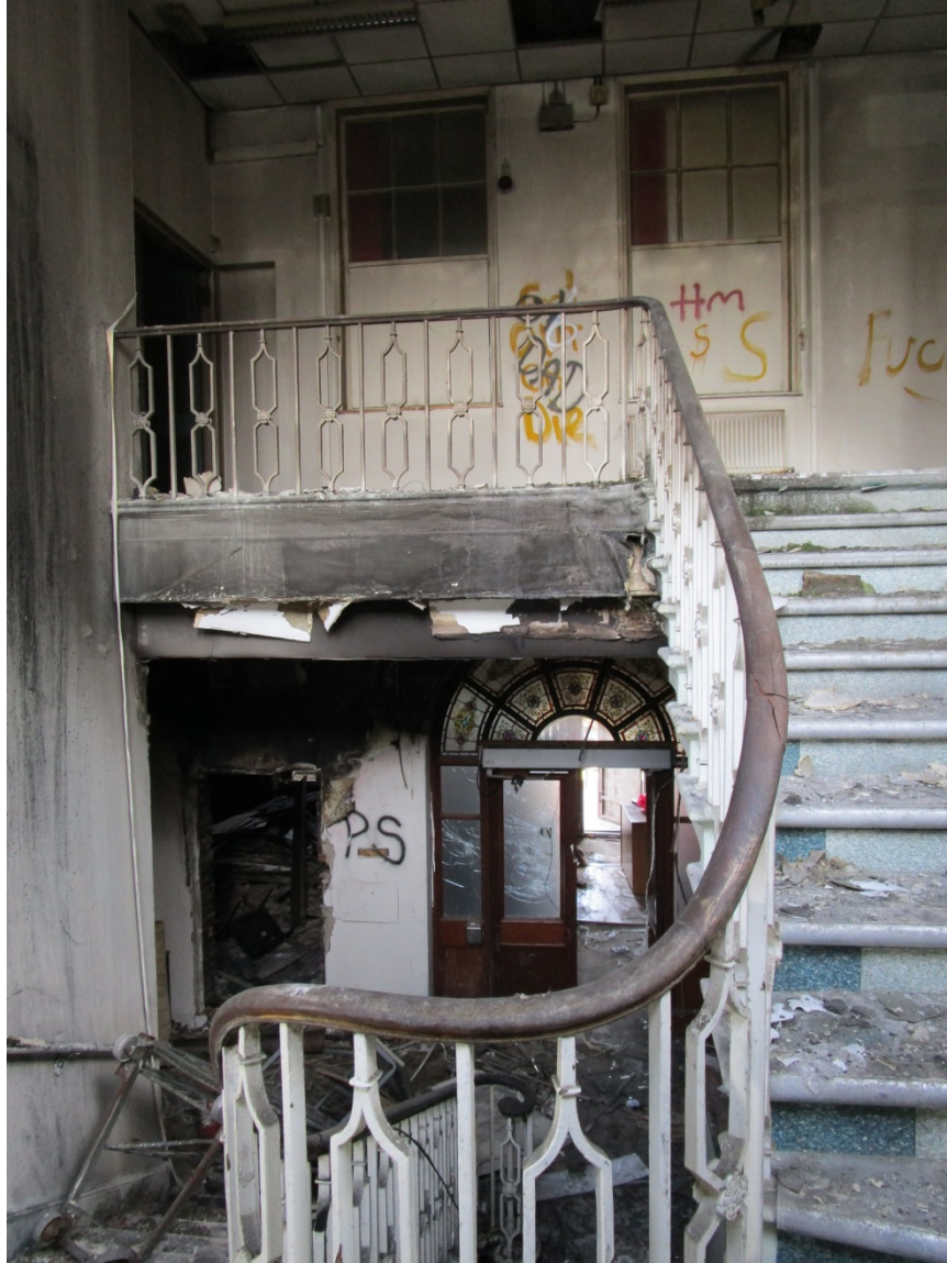
Plate 13: Stone cantilevered staircase in Block F1
