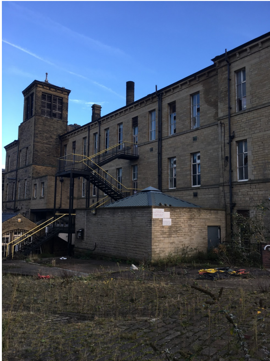
Plate 8: North elevation of the Carlile Wing (southern wing)
