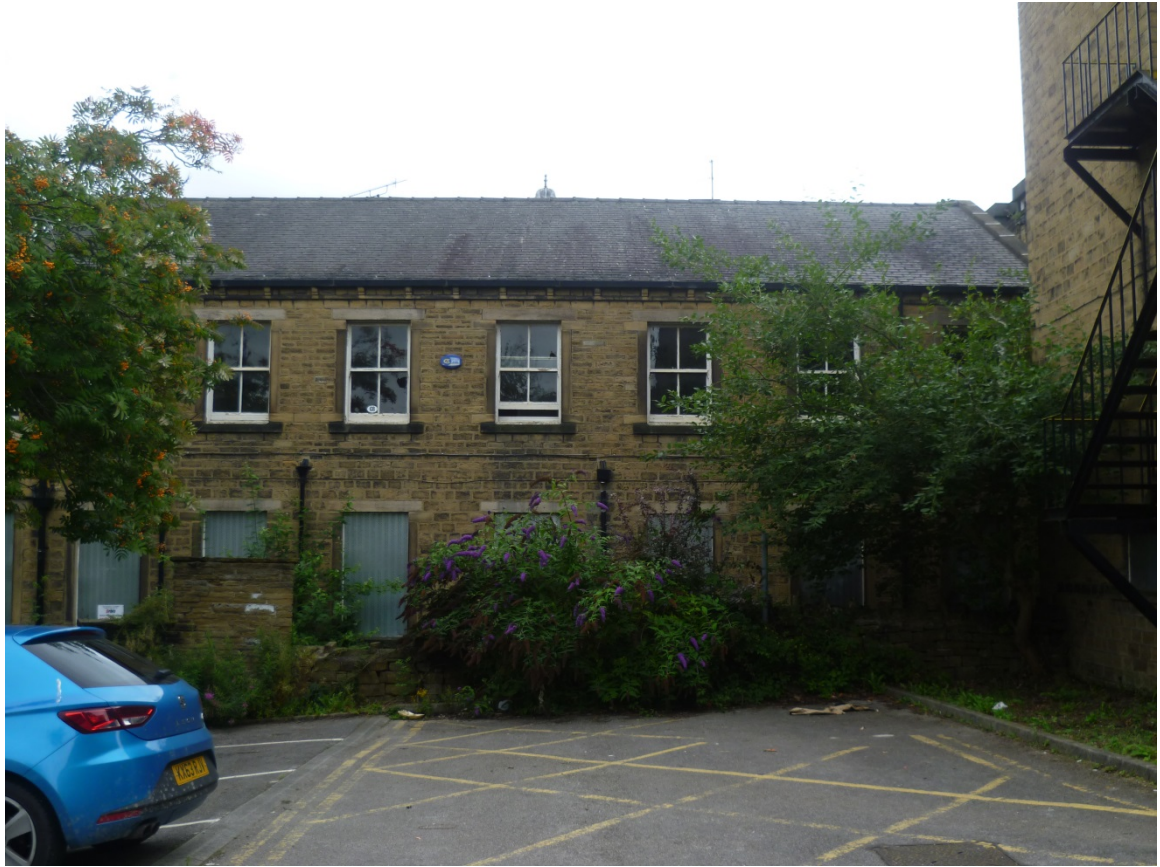
Plate 12: Block H2 north elevation
