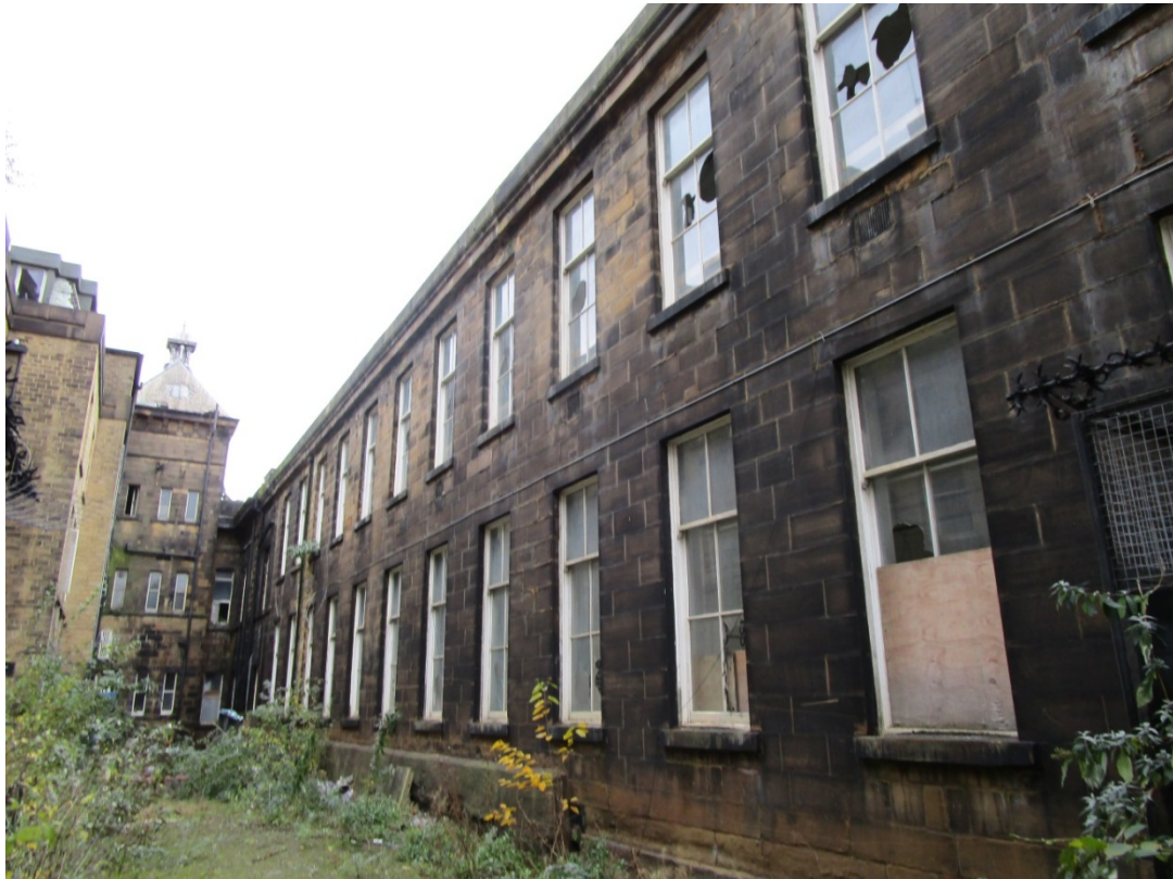
Plate 9: North elevation of the 1874 north wing extension
