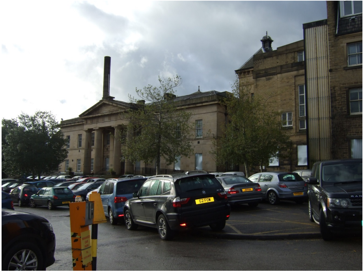
Plate 6: Front (east) elevation of the Infirmary building (Block F1)
