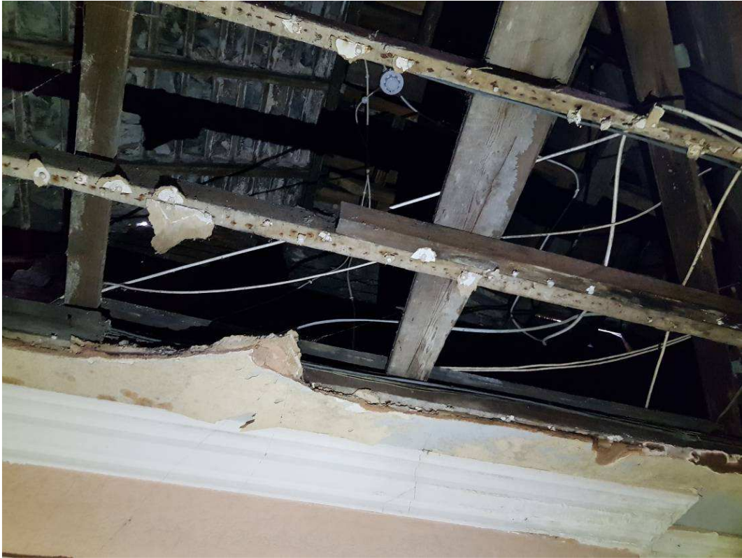
Photo 11: Internal view of loft timbers
