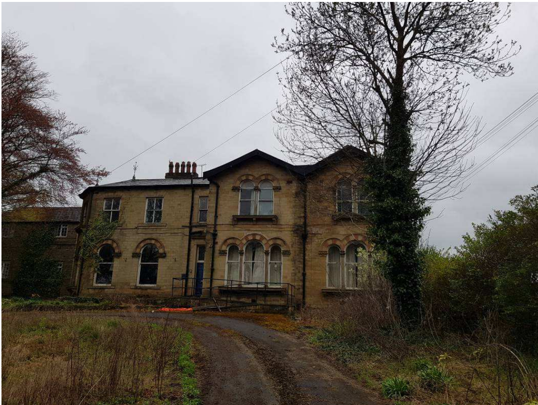
Photo 12: External view of main entrance to care home building
