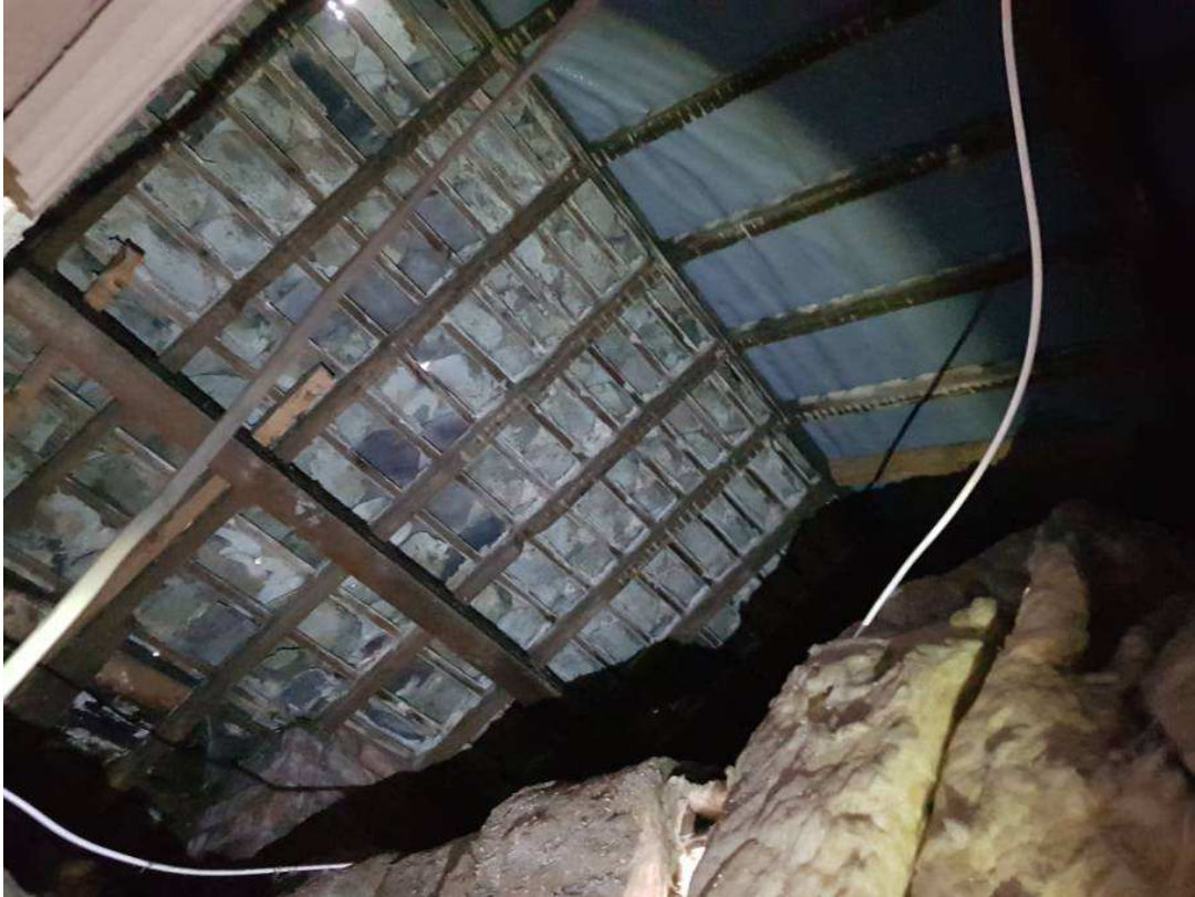
Photo 9: Internal view of ceiling, with fibreglass membrane present
