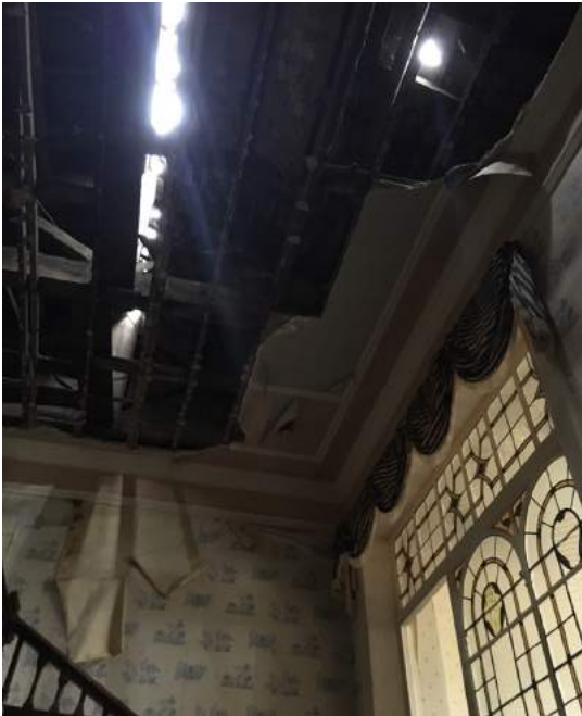
Views inside the vacant buildings
