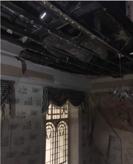
Views inside the vacant buildings
