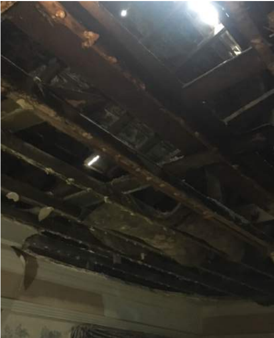
Views inside the vacant buildings
