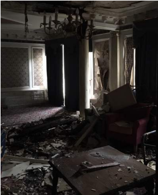
Views inside the vacant buildings
