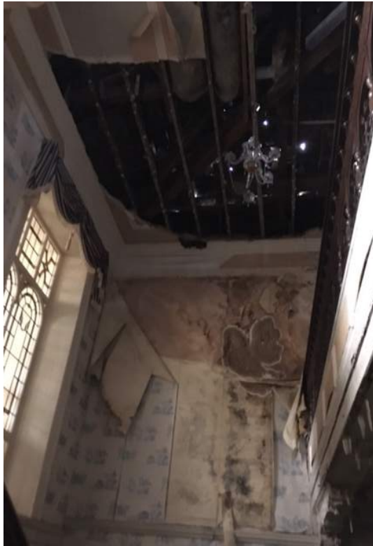
Views inside the vacant buildings
