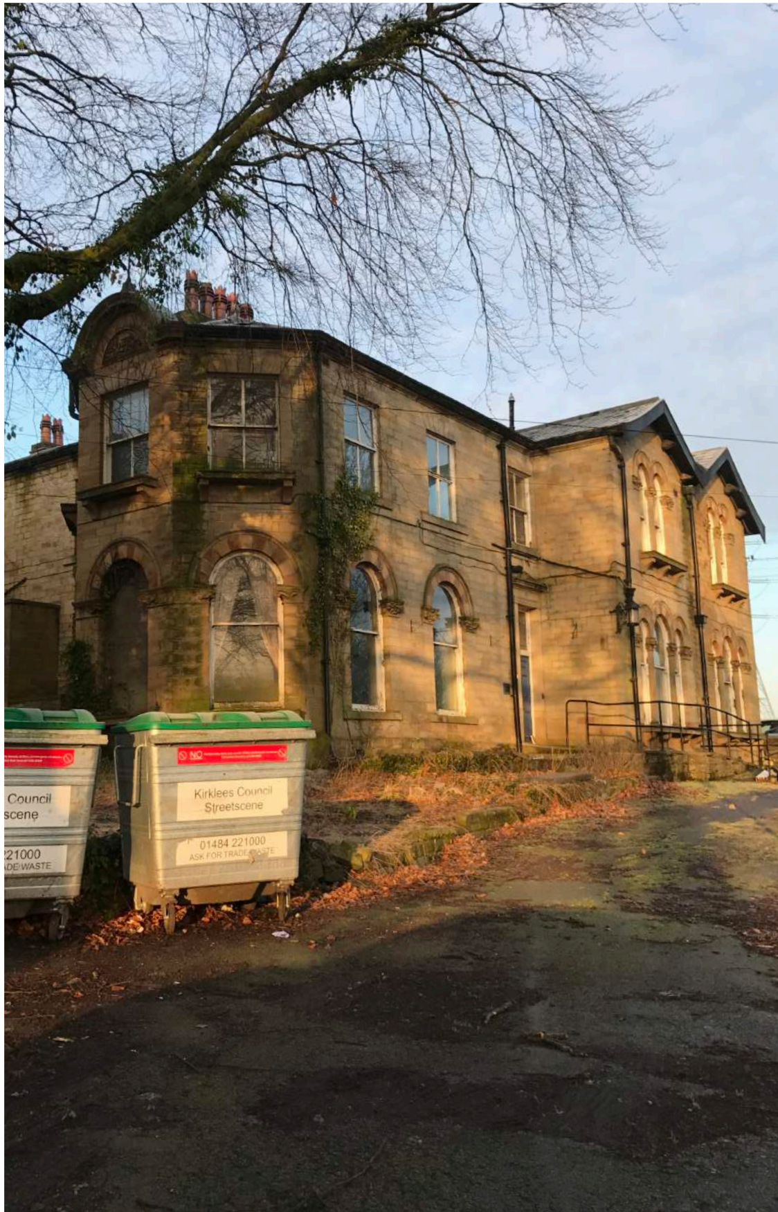
Front elevation to Holme House
