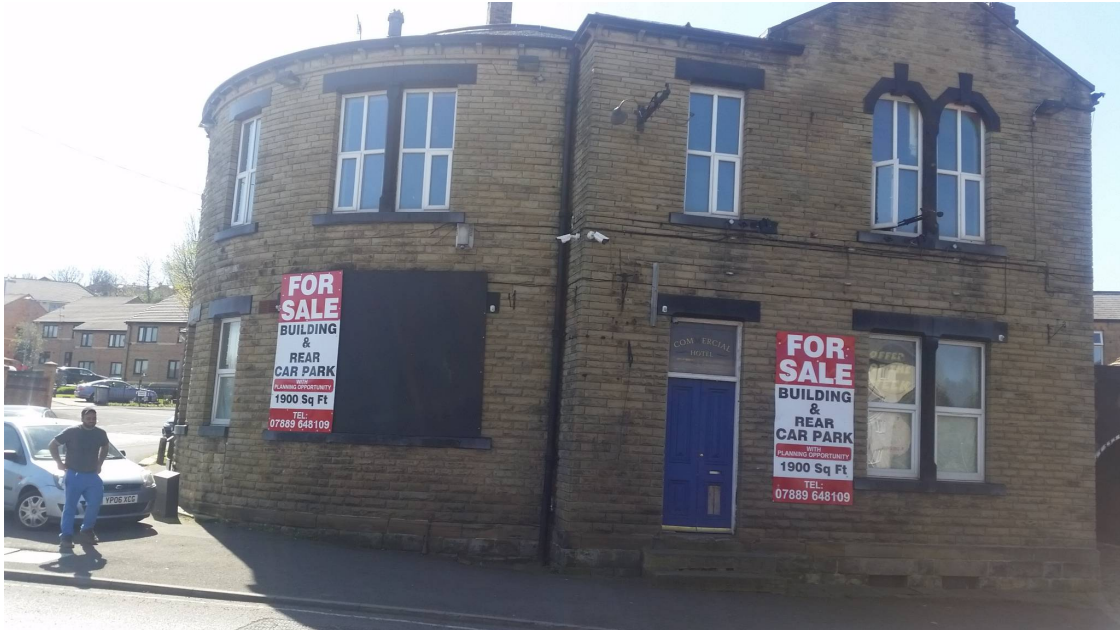
Picture 4: 125 Wellington Street is on a junction with Dark Lane.
