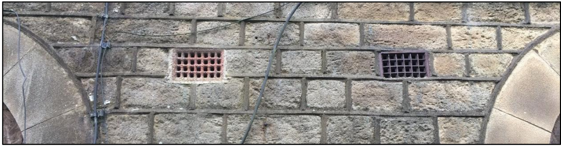
Internal inspection of fire station building
