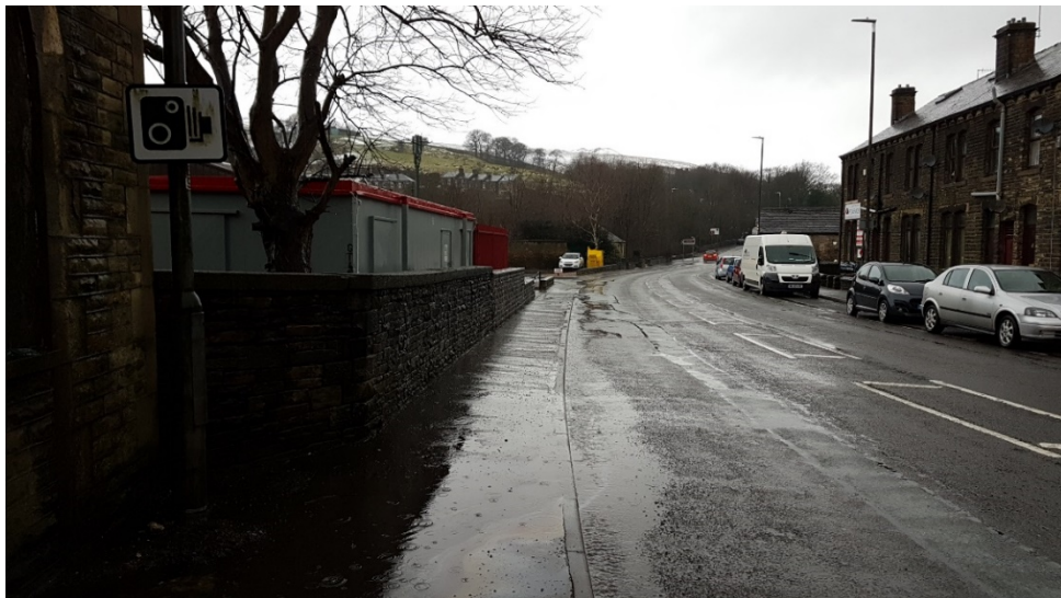
Photograph 2 – A62 Manchester Road Westbound
