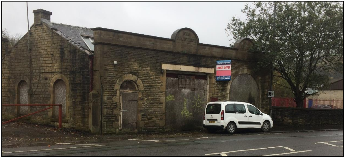
Plate 7. Rear of Fire station building (south elevation)
