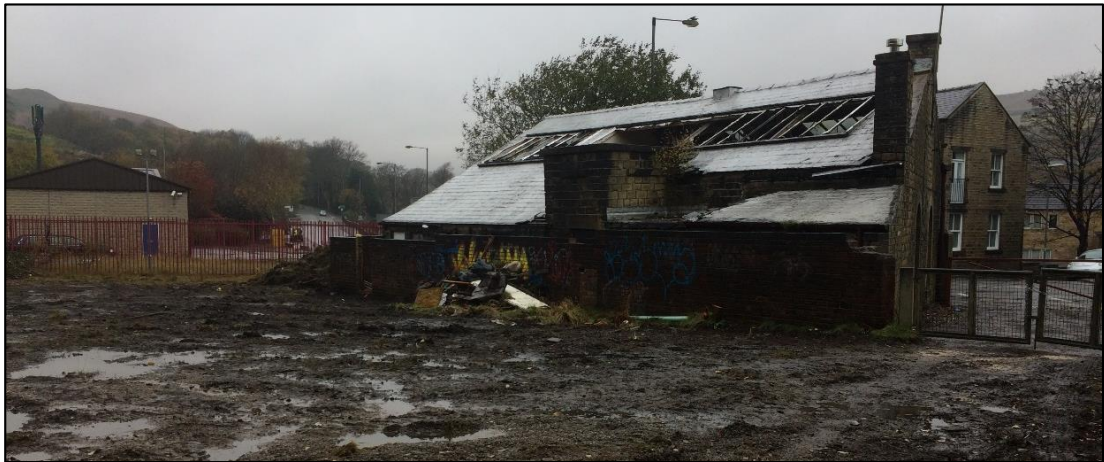
External inspection of fire station building
