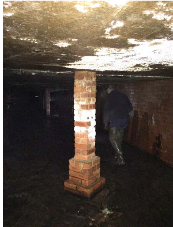
Brick piers, chainage 150
