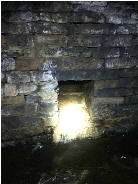
Incoming surface water culvert, chainage 30
