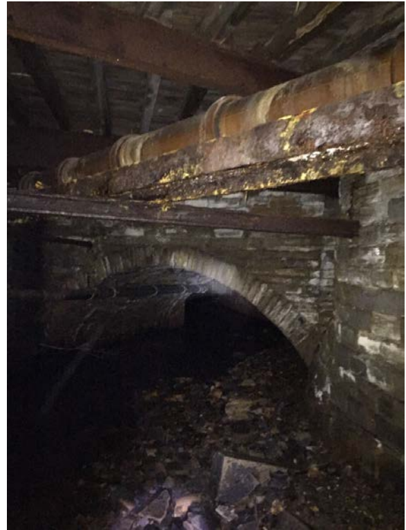
Remnant arch, chainage 13
