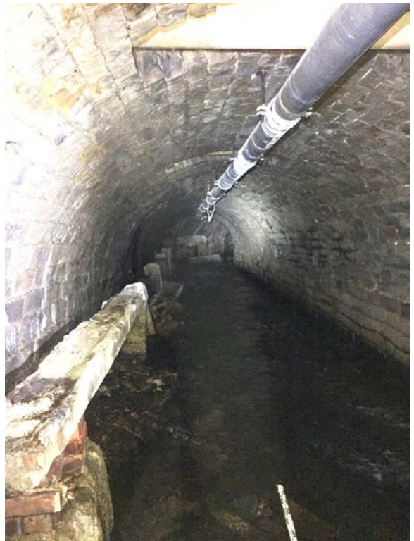
Barrel arch, upstream end of culvert
