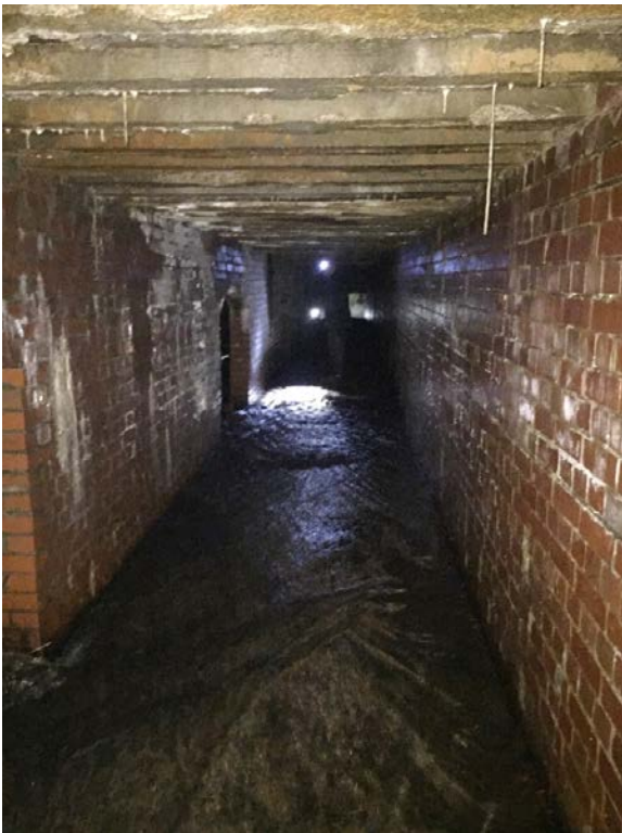
Brick arches, chainage 180
