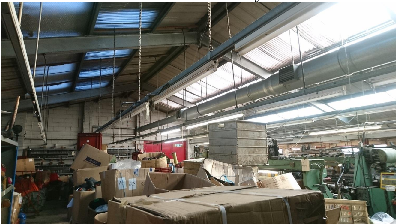
Photo 19: Internal view of Building 1.
