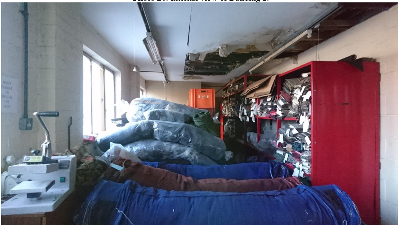
Photo 20: Internal view of Building 2.
