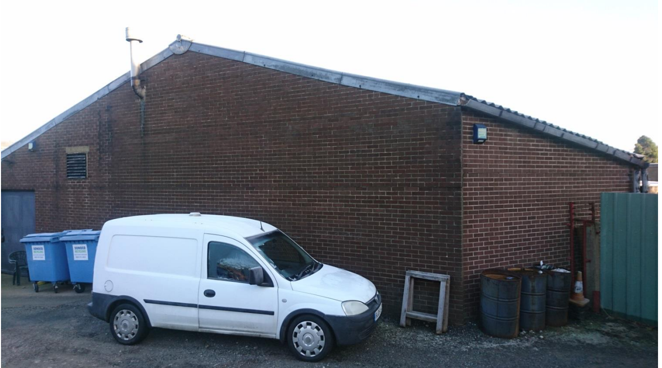
Photo 13: Building 1 looking northeast. Bat roost potential circled.
