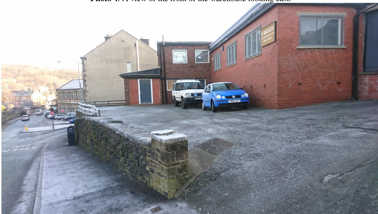
Photo 4: A view of the front of the warehouse looking east.
