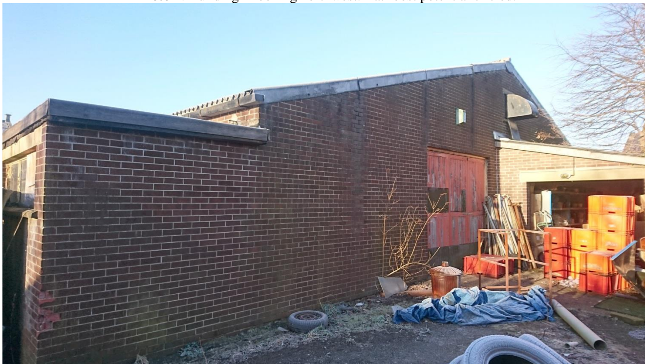
Photo 7: Building 1 looking northwest. Bat roost potential circled.
