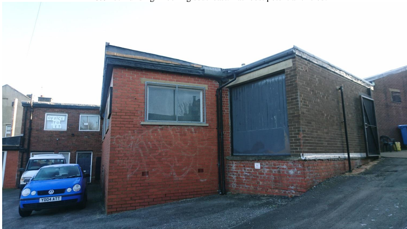
Photo 15: Building 2 looking southeast. Bat roost potential circled.
