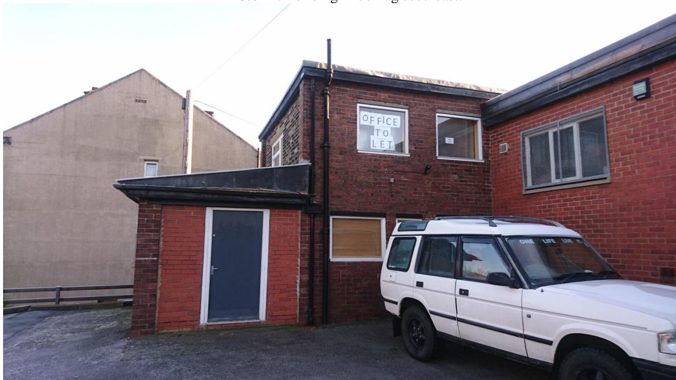
Photo 17: Building 2 looking southeast.
