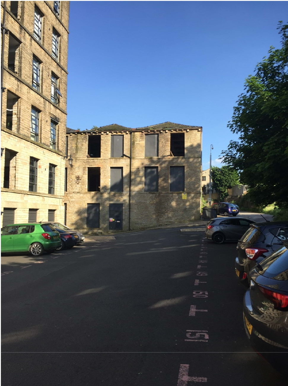
Existing Building Form 5
