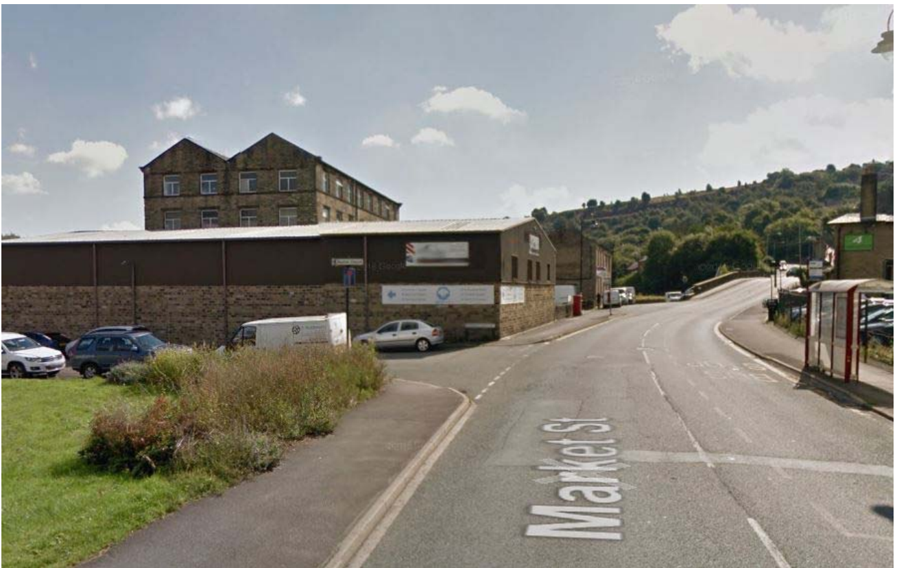
Existing Building Form 4
