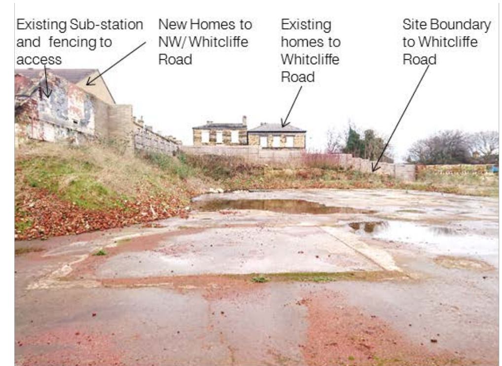
B : View outwards, to the North West of the site
