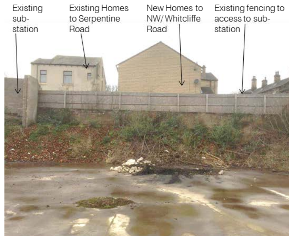
C : View outwards, to the West of the site
