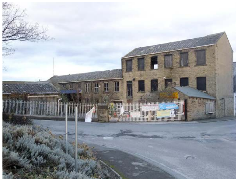
Views of now demolished mill buildings from Serpentine Road...
