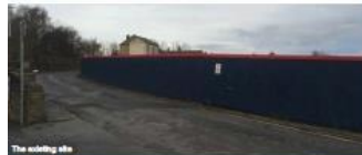
The existing site
