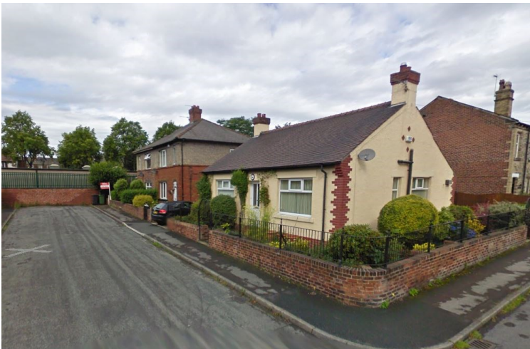
Brick and render bungalow and houses to rear of site off Bramhope Road
