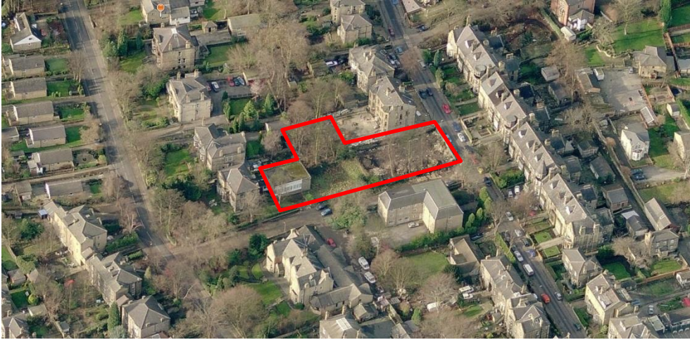
Image 01: Aerial view of the site
