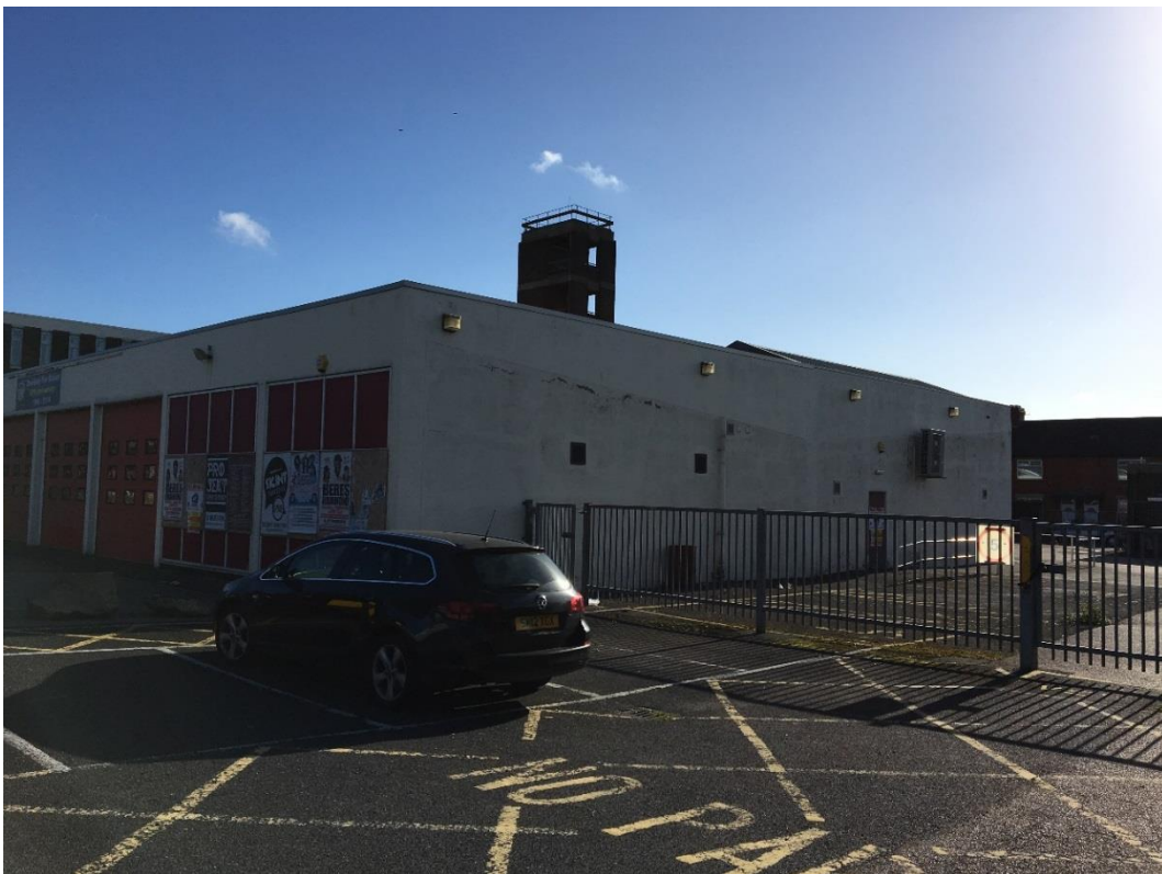
Figure 3: Ancillary accommodation to appliance bays
