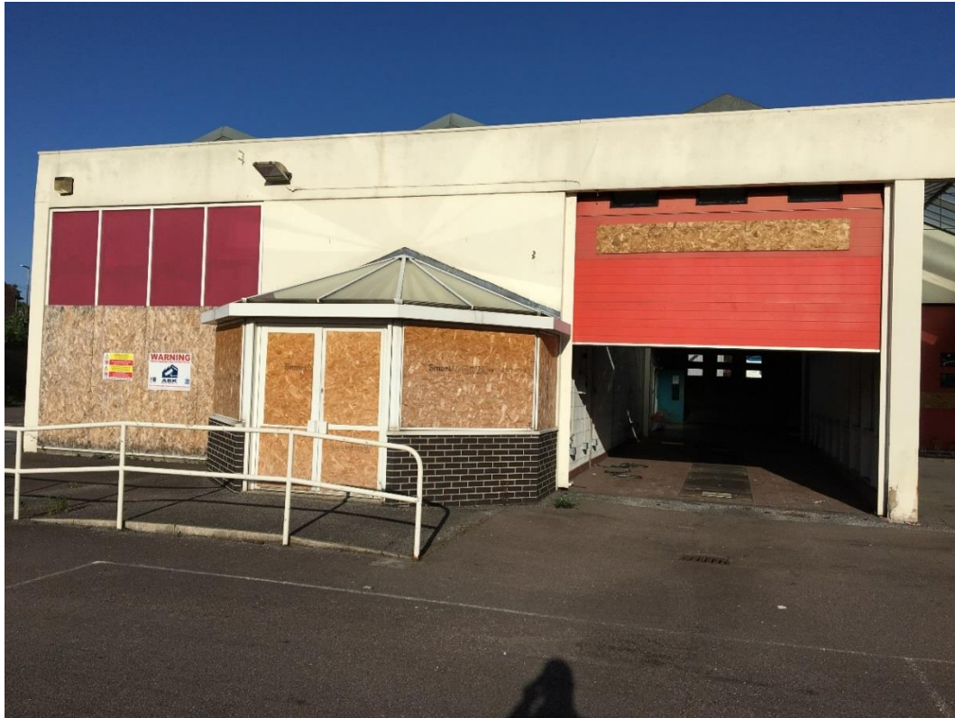
Figure 4: Ancillary accommodation to appliance bays
