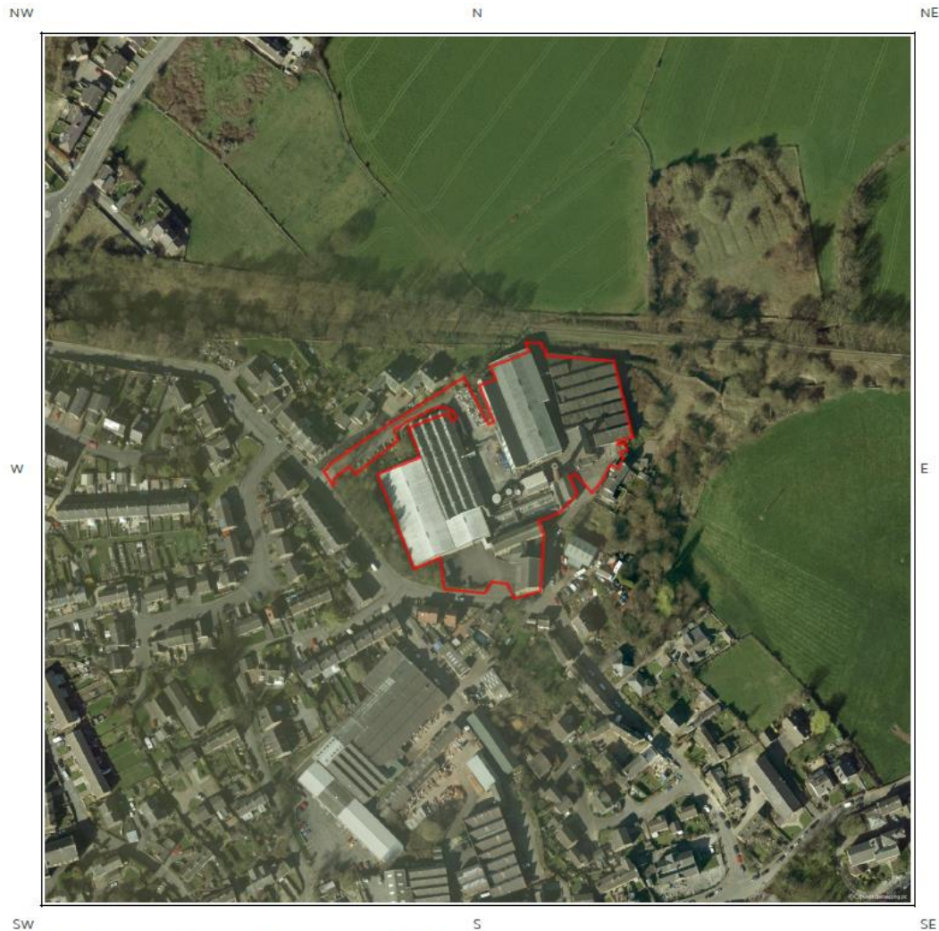
Aerial Photograph Capture date: 26-Mar-2012 Grid Reference: 423372,410949 Site Size: 1.18ha
