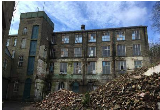
3 – Existing Mill building
