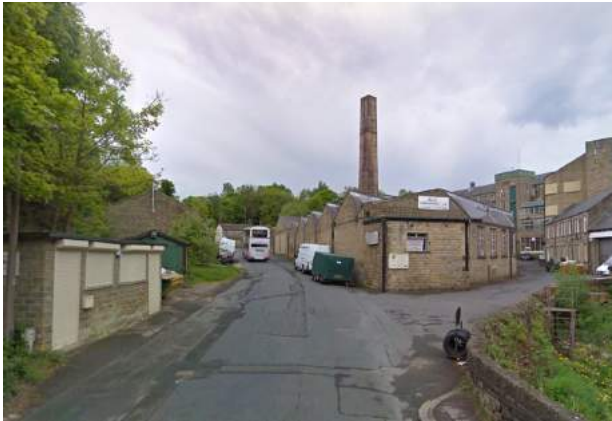
1 – Existing Mill Access from Hepworth Road
