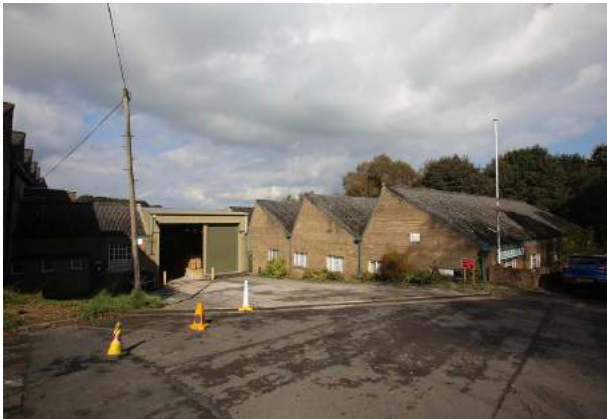
2 – View of existing mill buildings from car park
