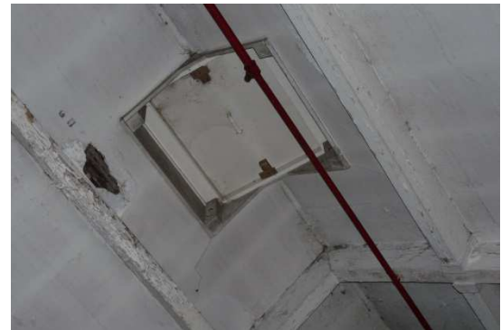
Access to ridge vents
