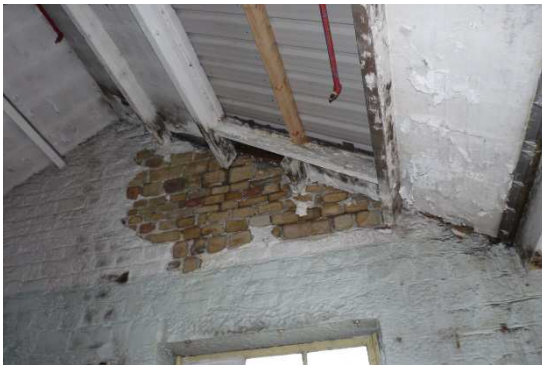
New roof sheeting
