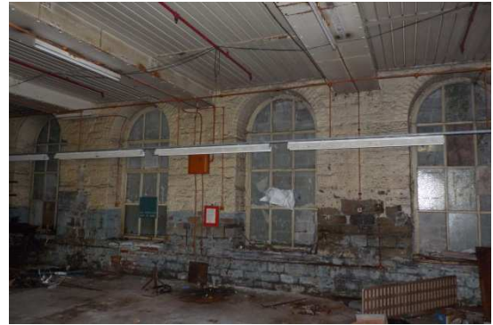
View of the south west corner; pairs of steel beams under the 1 st floor
