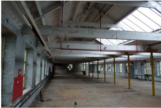
Timber roof trusses
