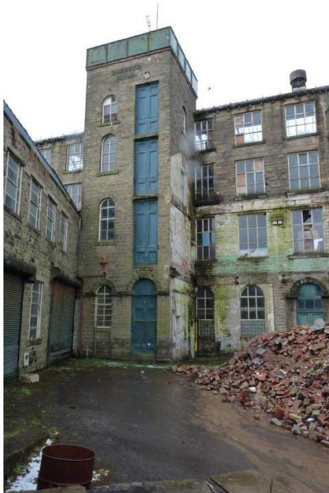
External staircase with water tank at the top
