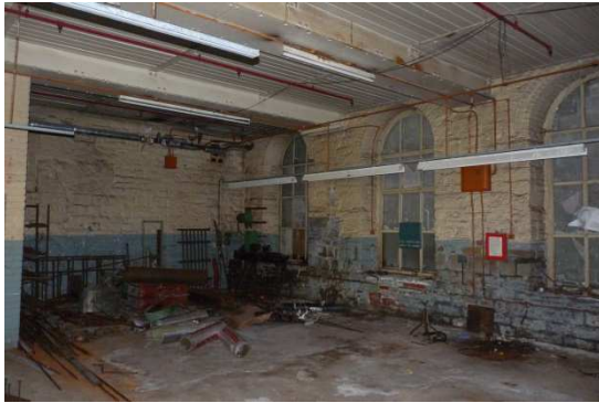
View of the south west corner; pairs of steel beams under the 1 st floor
