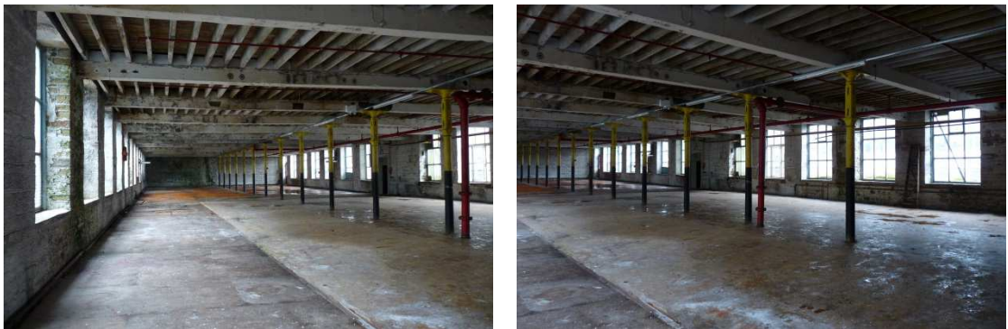
Views looking towards the north gable
