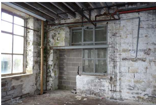
Alterations to the south gable wall window
