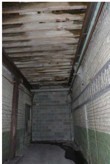
Blocked up entrance arched
