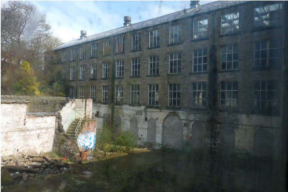
Rear view of the mill (southeast elevation), previous ground level extensions now demolished
