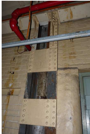
Additional steelwork strengthening
