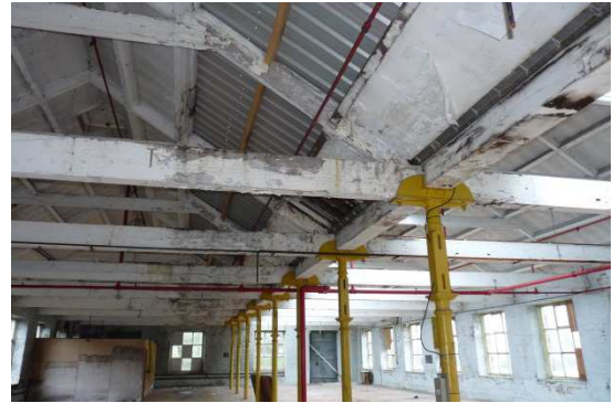
Central valley and new roof sheeting
