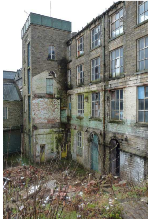
Lean-to extension now demolished
