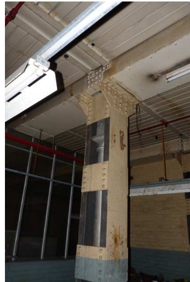
Additional steelwork around a column
