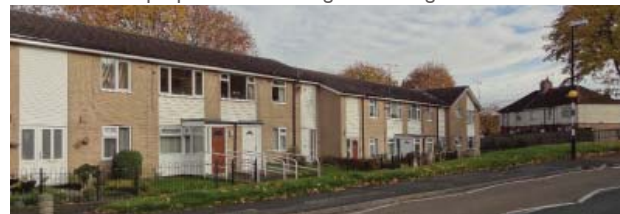
Front elevations over looking Lees Hall Road.
