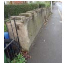
Boundary Treatment: Mainly walled boundaries of either brick or concrete. Between plots some low metal fencing but this does vary
