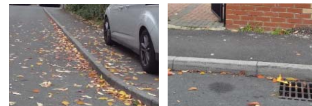
Surface Treatment: Both the pavements and the roads are made up of tarmac with concrete curb stones defining the pavement edge
