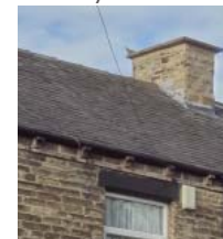
Roofing: The roof material on the older properties are slate, the newer buildings could be artificial slate
