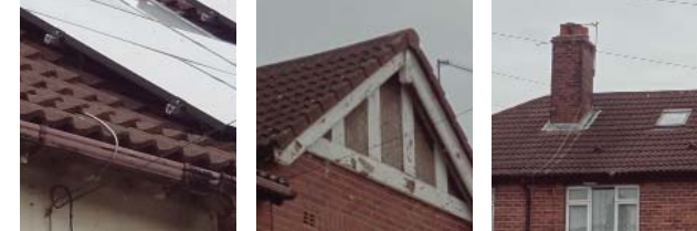
Roofing: Original tiles are profiled red clay pantiles. Gables articulate mid terraces or bookend end units. Some solar panels are in evidence.
