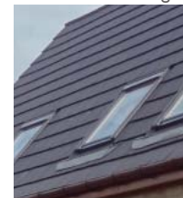
Roofing: The roof material on the older properties are slate, the newer buildings could be artificial slate
