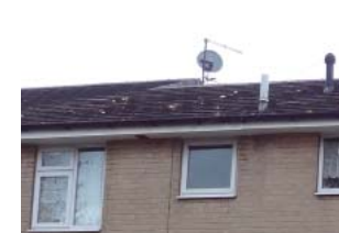
Roofing: Low pitched dual pitched roof with shallow eaves
