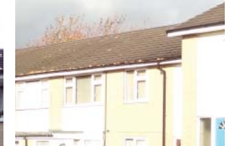
Roofing: Low pitched dual pitched roof with shallow eaves
