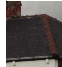
Roofing: Slate, clay or concrete roof tiles. Steeply pitched, hipped roof with deep eaves and central chimneys
