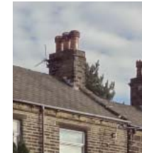
Roofing: Slate roofs pitched front to back with chimneys halfway down the roof. Shallow eaves with brackets and fascia boards tight above lintel
