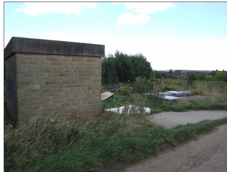
Plate 6. View of small brick building in the centre of site, looking north-east
