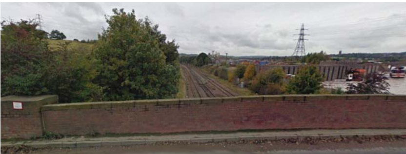
50. Ravensthorpe rail bridge
