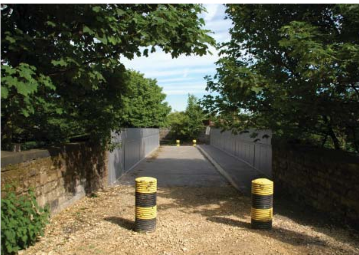
43. Footbridge over railway
