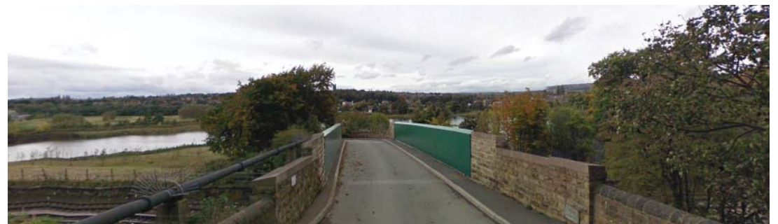
31. Sands Lane rail bridge
