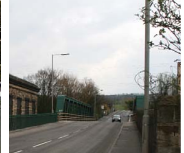
49. Calder Road river bridge
