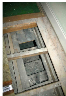
Floor boards beneath the stairs at first floor level removed to reveal existing original timber stair from first to ground floor
