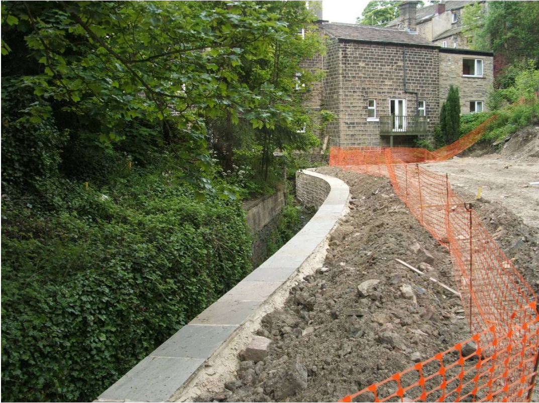
Photo – 5 Improvement works to west side of watercourse open channel
