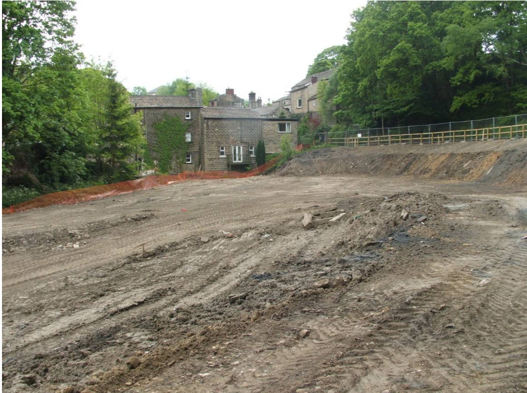
Photo 7 – site clearance to south of site, open channel to the left of picture
