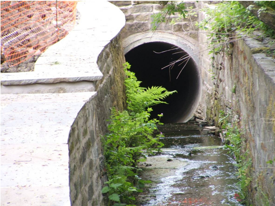
Photo 6 – New entrance to culvert
