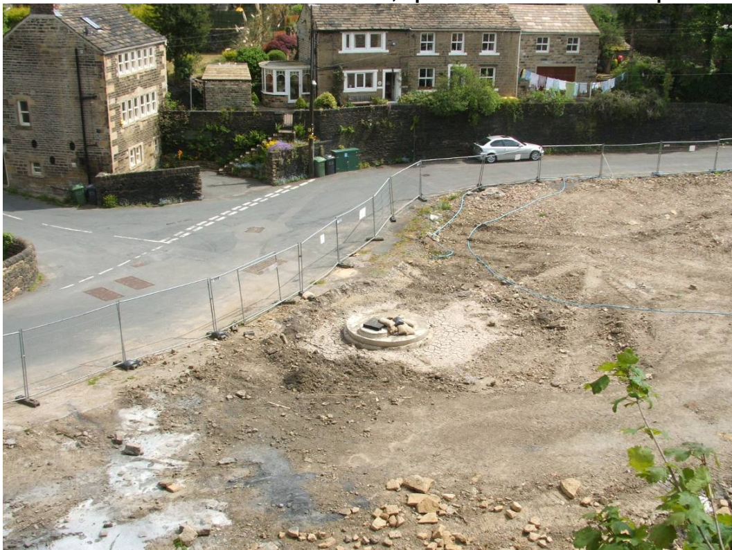
Photo 8 – site clearance to north of site showing new culvert manhole. Culvert continues under Thirstin Road to the left for approximately 30 metres
