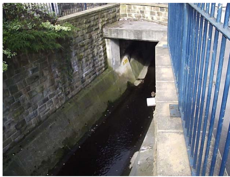
Figure 4.1: Downstream end of Batley Beck culvert.
