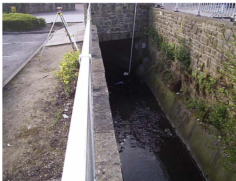
Figure 4.2: Upstream end of Batley Beck culvert.
