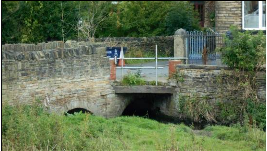
Figure 4: Cliff Hollins Lane road bridge at Oak Mills - downstream
