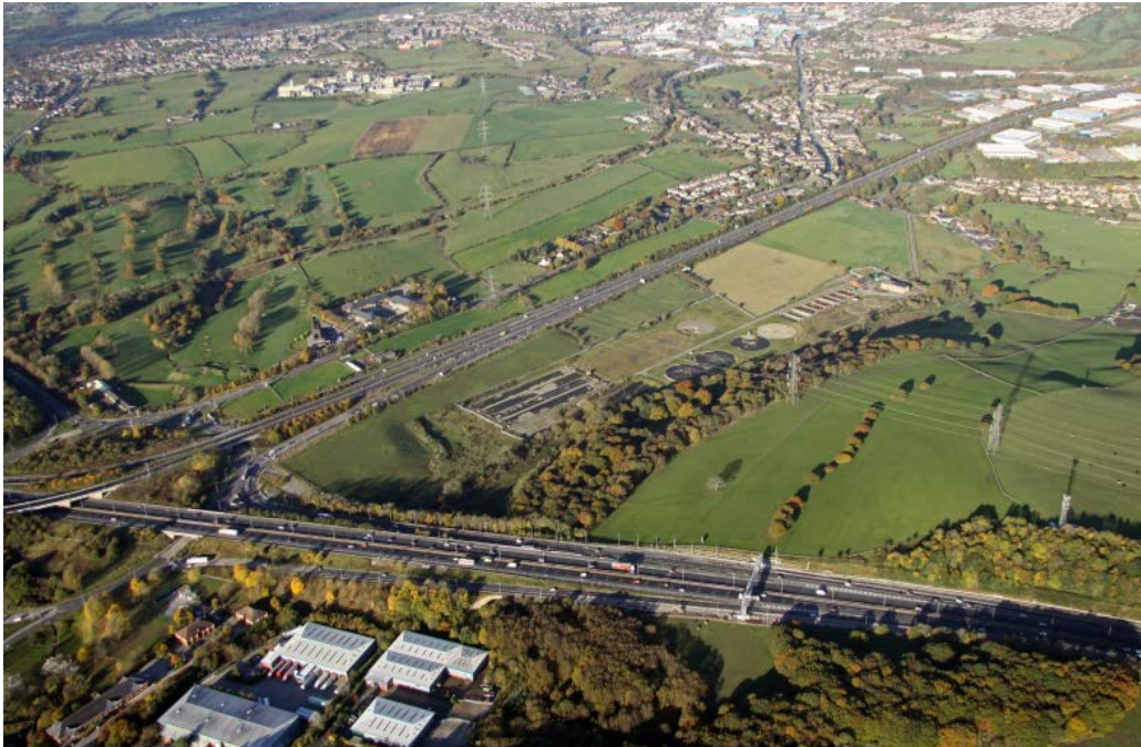
Figure 2: Aerial photograph of the site looking north-west towards Oakenshaw, Euroway and Low Moor
