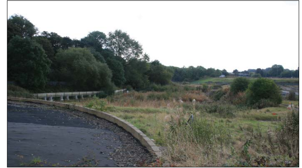
Plate A7.24: Settlement Tanks
