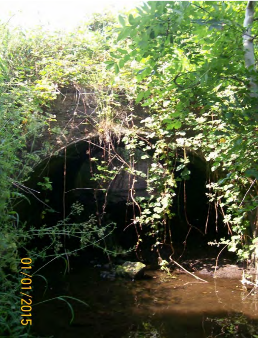
Stone Arch Culvert (XS33.5)
