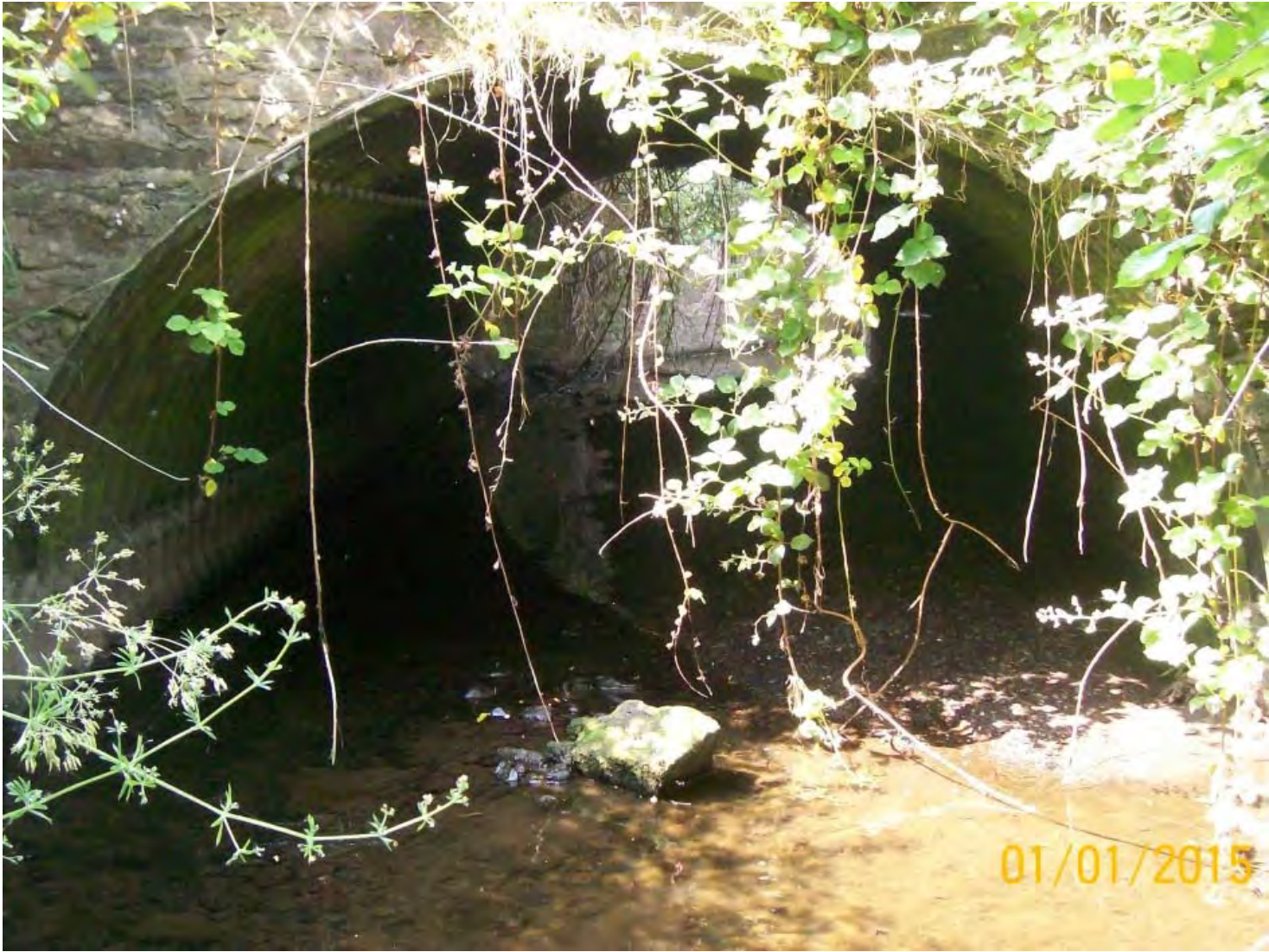
Stone Arch Culvert (XS33.5)
