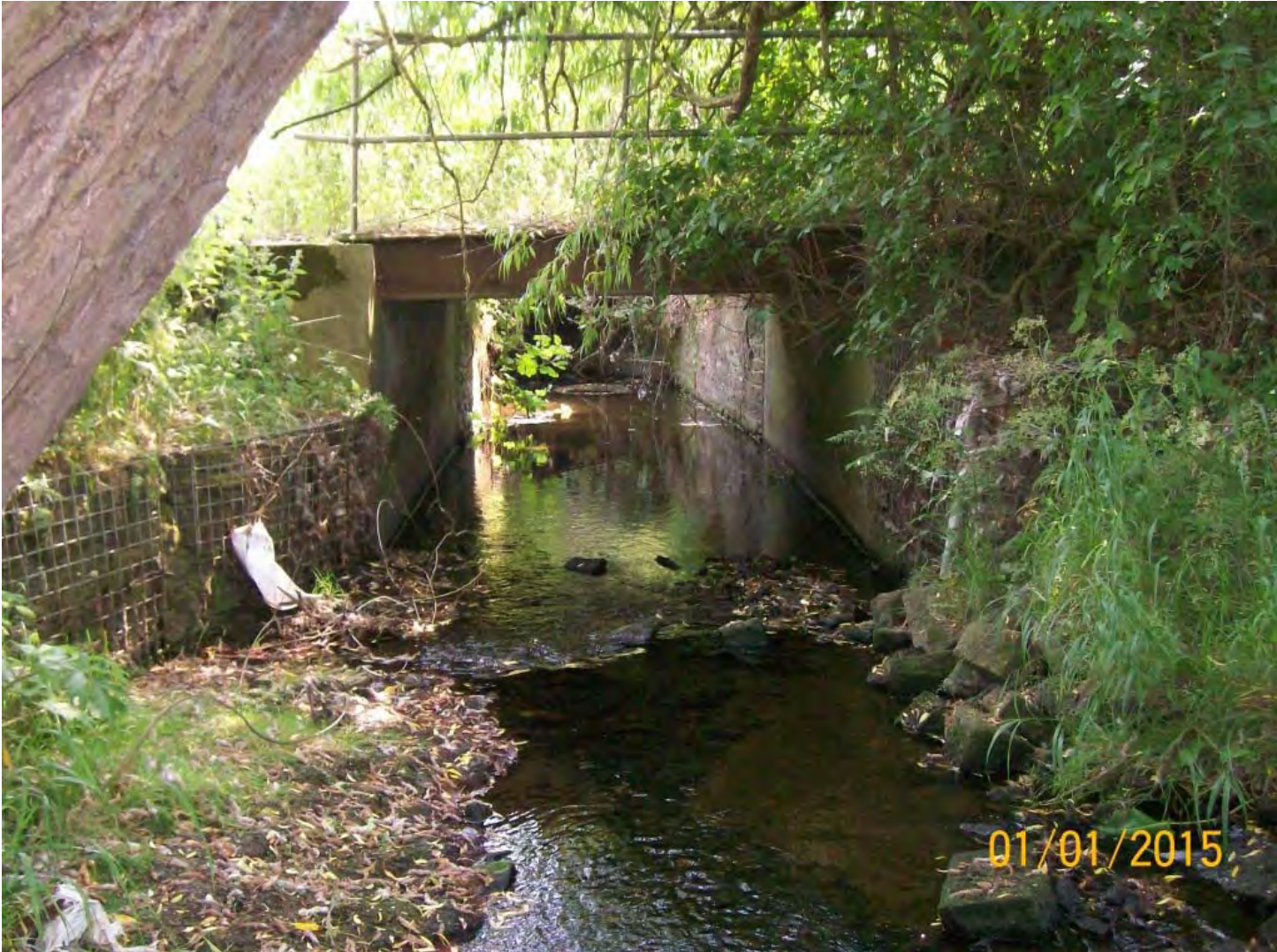
Vehicular Bridge (XS35.5)
