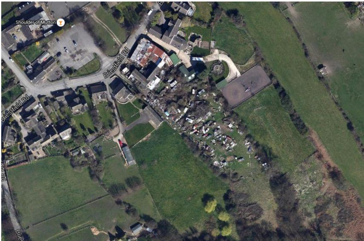
Figure 4- Site, currently used as a scrap yard
