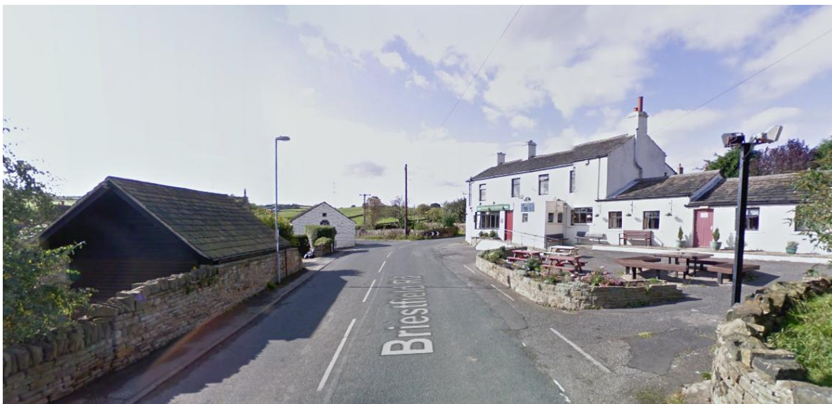
Figure 10- Neighbouring rendered building opposite the scheme at Poplar Farm.
