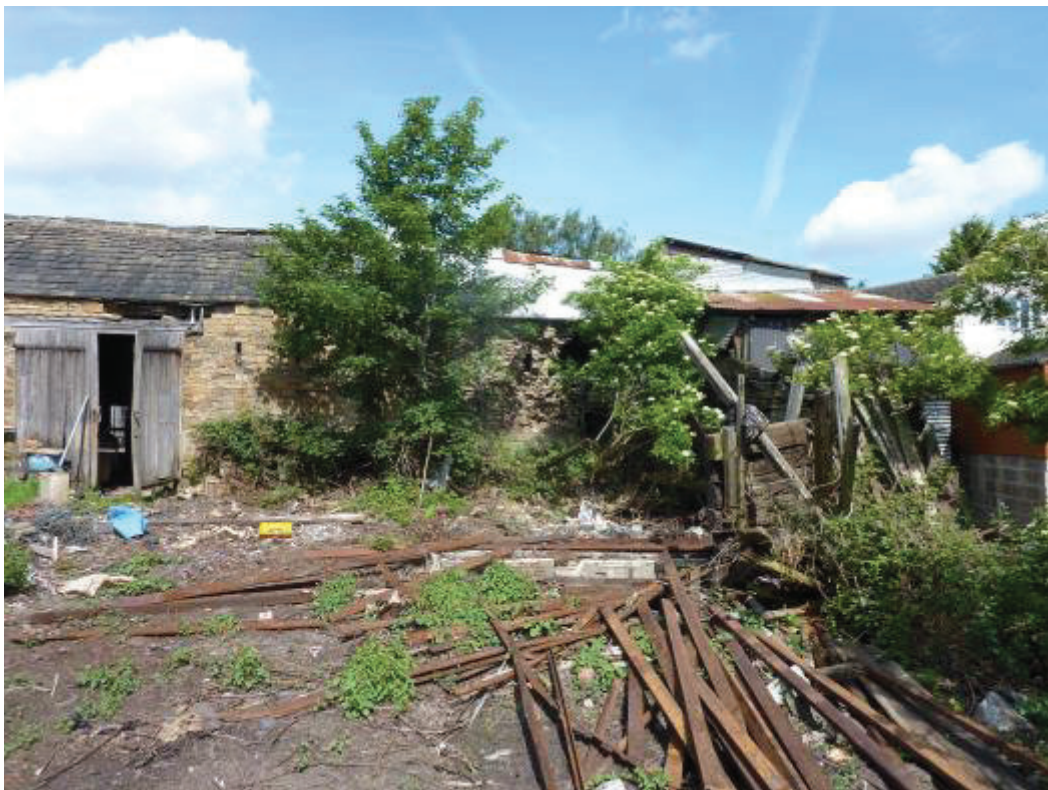
Photo 8: South elevation of barn & connected sheds
