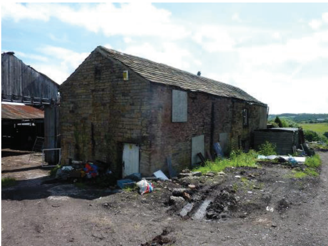
Photo 2: Northwest elevations of farmhouse.
