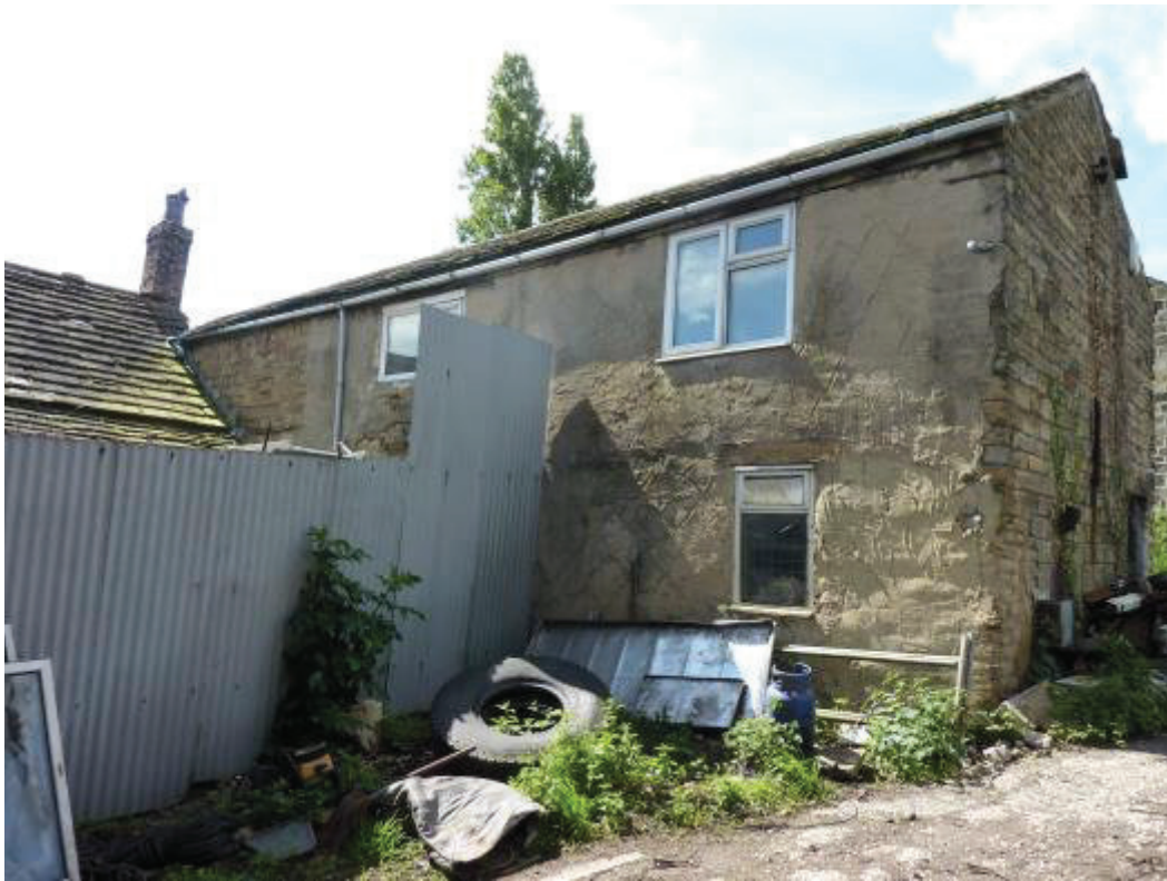
Photo 3: East elevations of farmhouse (stone barn to left of photo).
