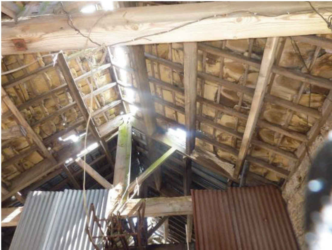
Photo 9: Light levels within Stone barn
