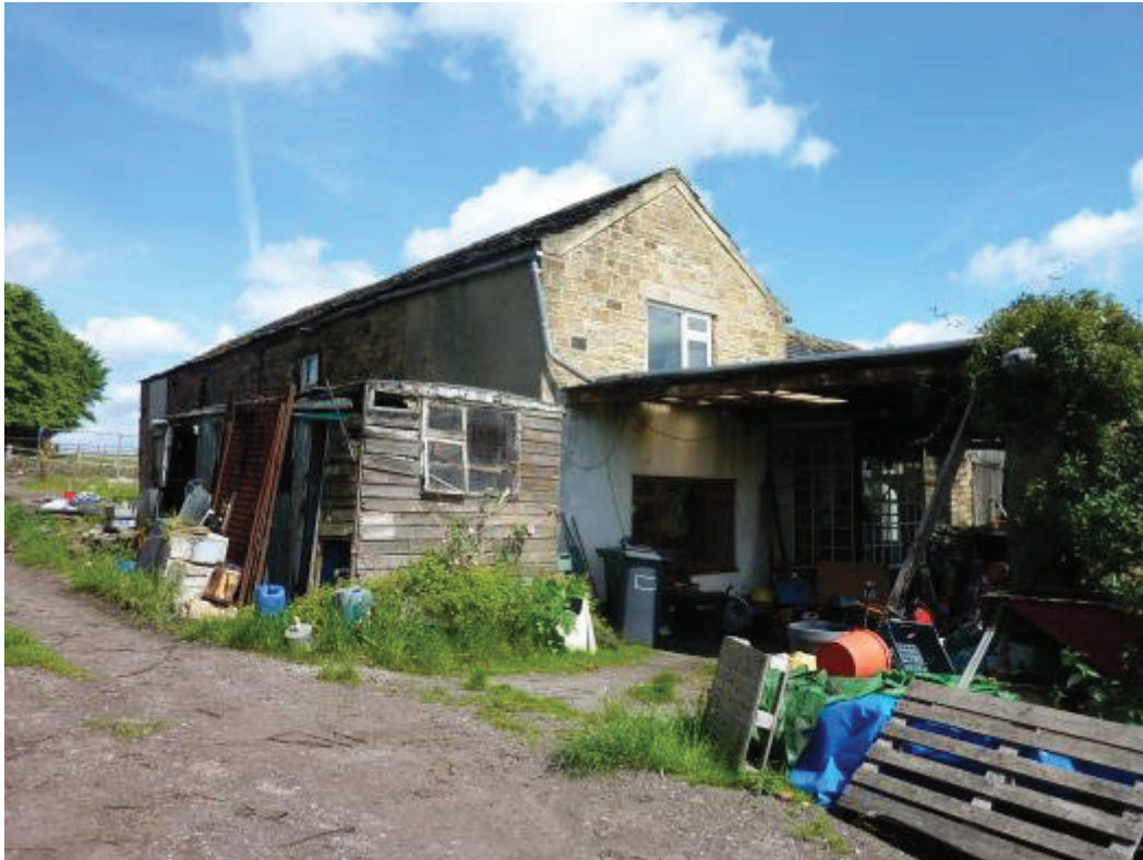
Photo 1: Southeast elevation of farmhouse.
