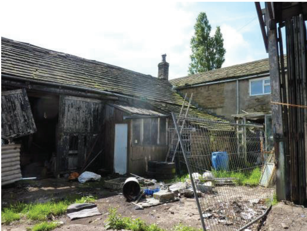
Photo 4: North elevation of stone barn.
