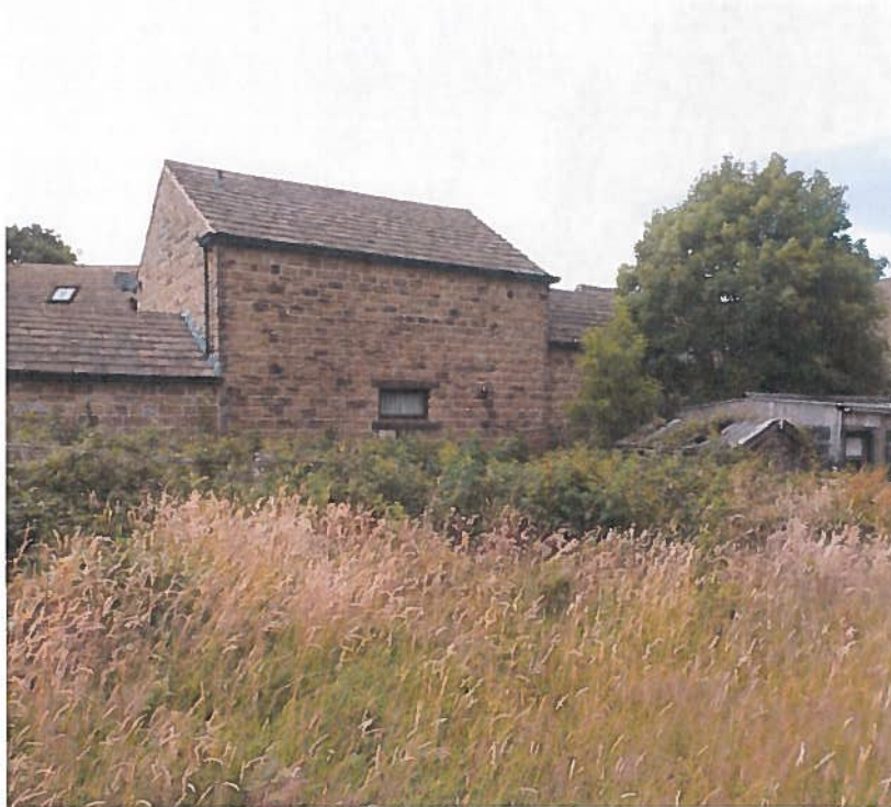
Figure 10: View towards the north west boundary.
