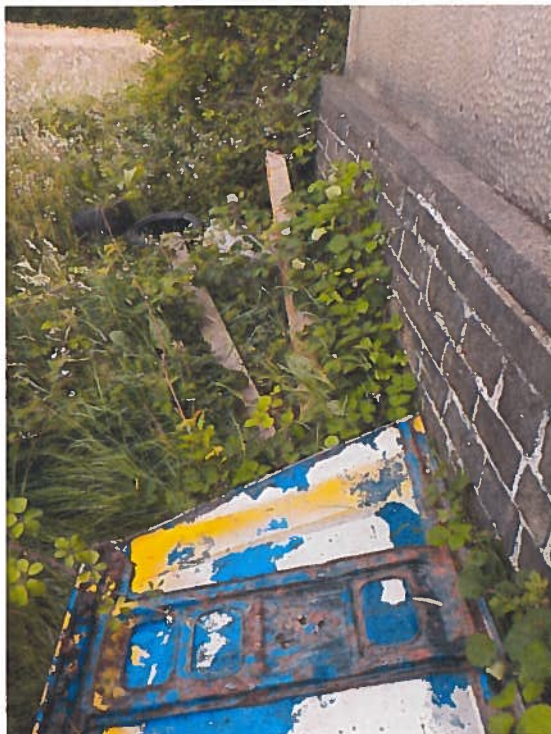
Figure 8: Car bonnet, timber and tyres in southern corner of site.
