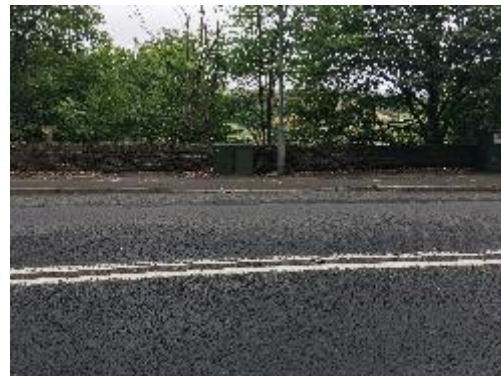
A62 Manchester Road – BT Cabinets / dropped crossing
