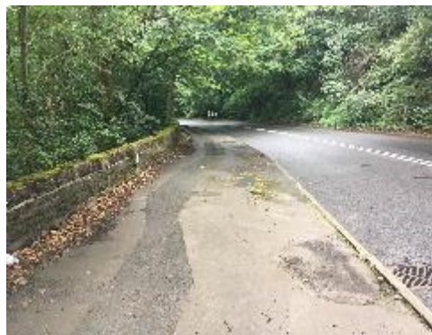
A62 Manchester Road east of access road
