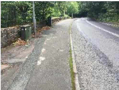
A62 Manchester Road looking East
