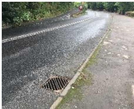
A62 Manchester Road west of access road
