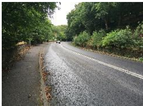
Double white line system on A62 Manchester Road looking East
