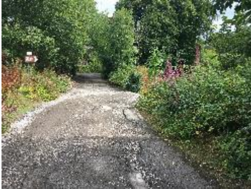
Access Road at J/W Entrance to Healing Centre
