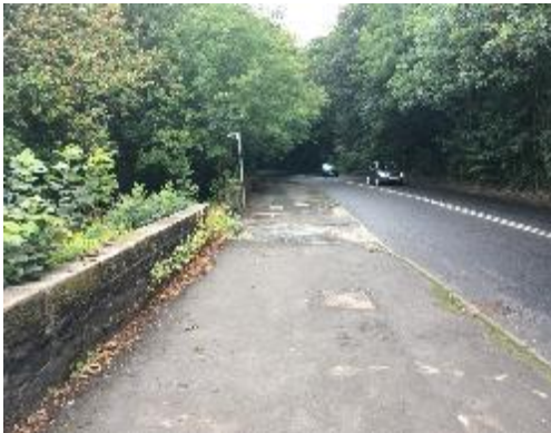
A62 Manchester Road looking towards access road.
