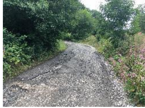
Access Road approaching bend
