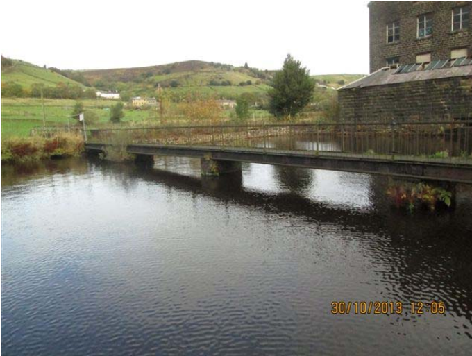
25. Footbridge over d/s (east reservoir)
