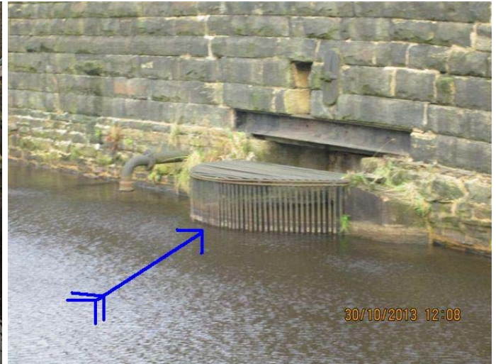
26. Outlet into mill building
