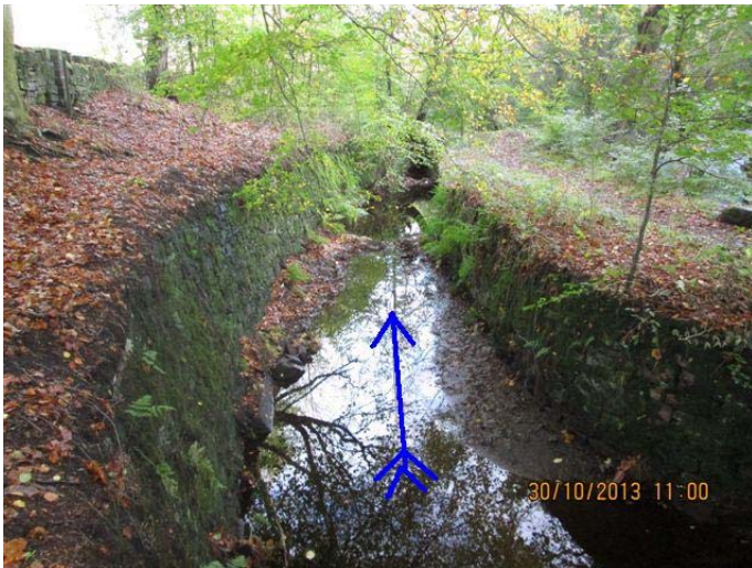
3. Masonry lined inlet channel
