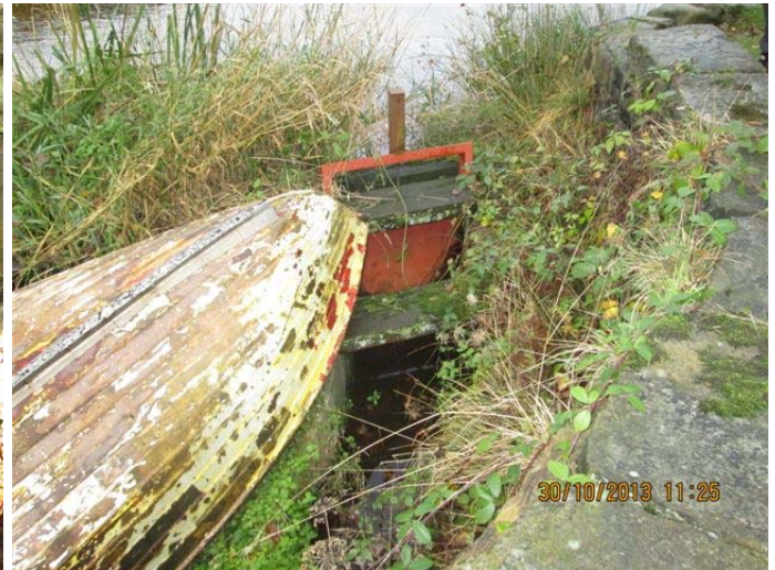
10. Sluice control on left side of overflow
