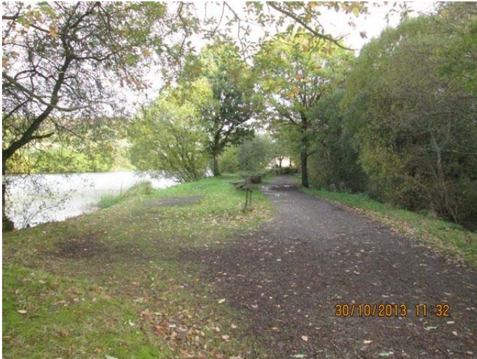
13. View looking north east across crest
