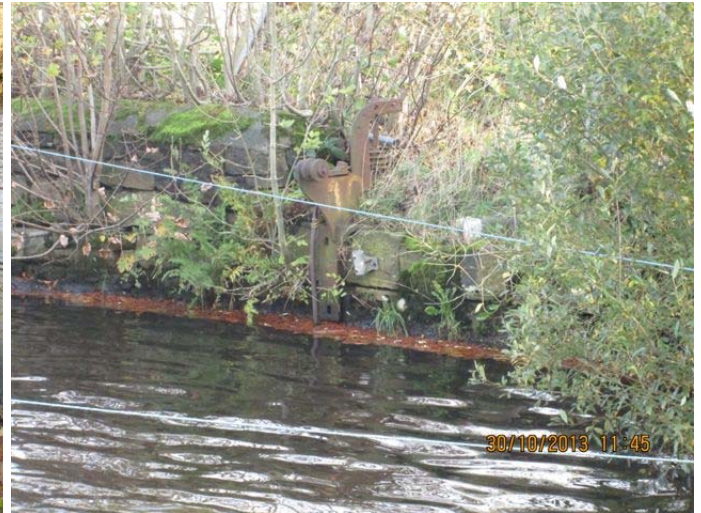
20. Sluice control in intermediate dam.
