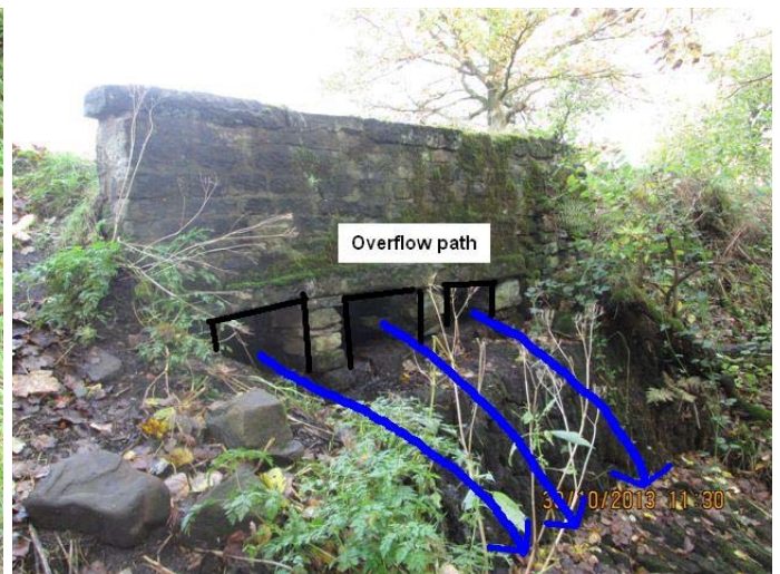
12. Culverts from overflow into watercourse
