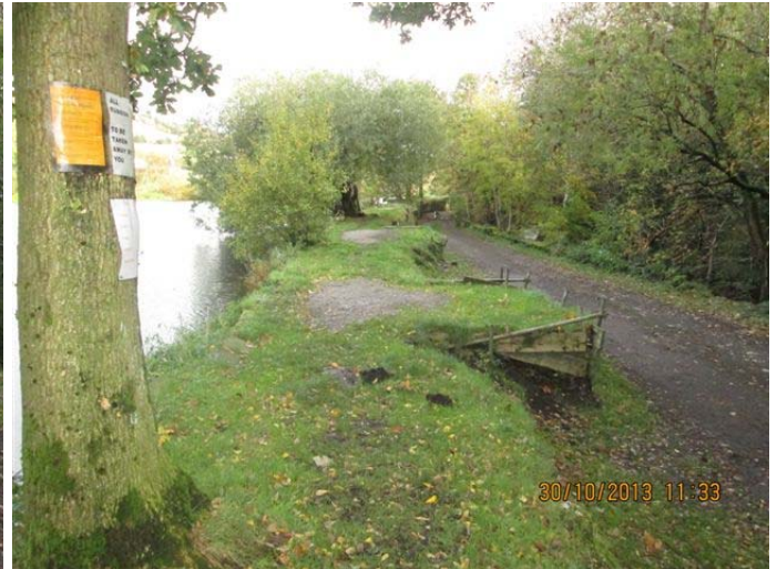
14. View looking north east across crest
