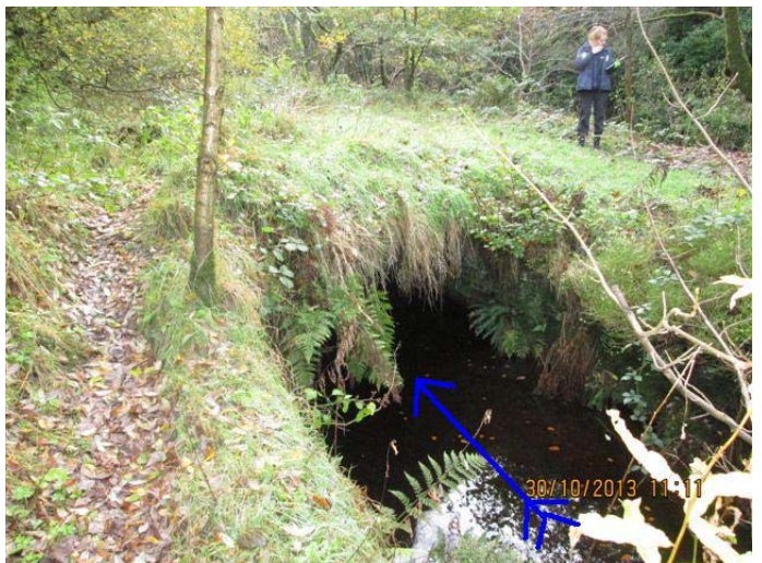
6. Bridge over inlet channel
