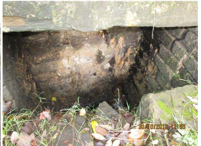
22. Chamber in masonry retaining wall
