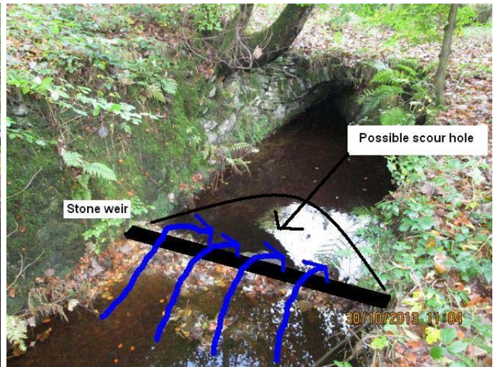
4. Stone weir in inlet channel
