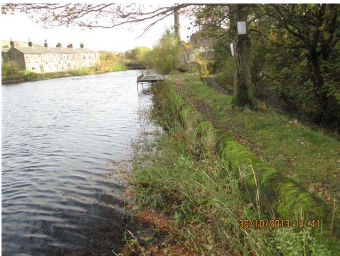
17. View looking east across upstream face
