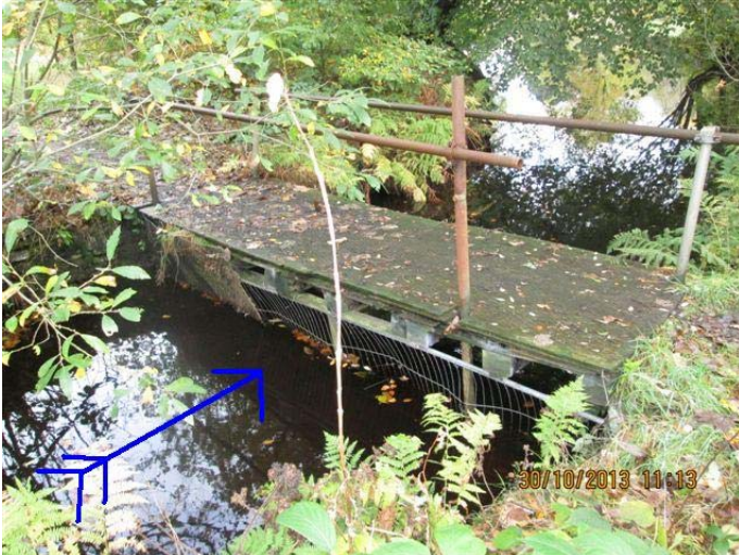
7. Scaffold access bridge over inlet channel
