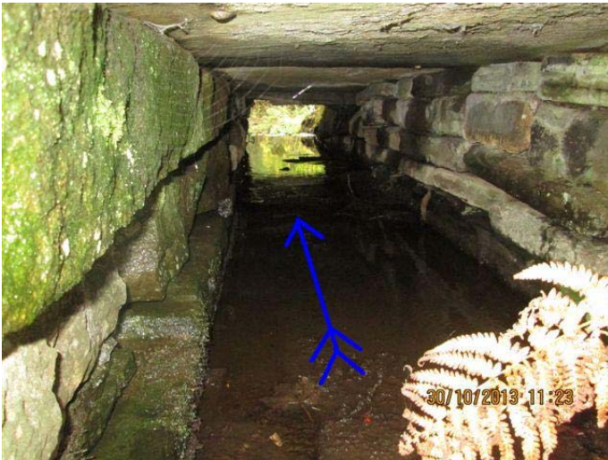
9. Rectangular culvert from overflow
