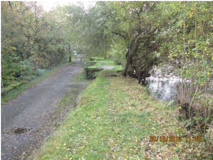
15. View looking south west across crest
