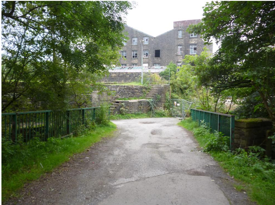
Photograph 1 – Existing Mill Buildings
