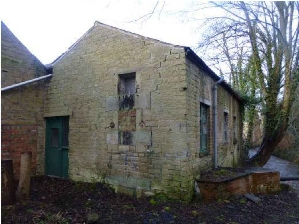
Photo 6: Building 2 viewed from the south-east (watercourse visible on right)
