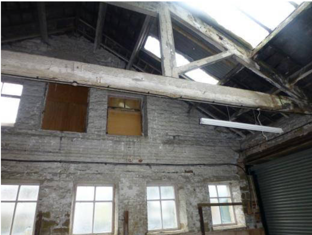
Photo 7: Internal roof structure of Building 2
