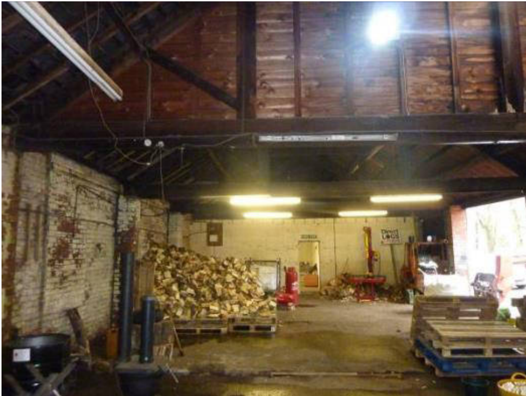
Photo 4: Internal of Building 1
