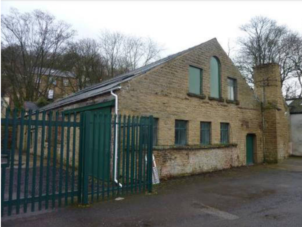
Photo 5: Building 2 viewed from the north-west
