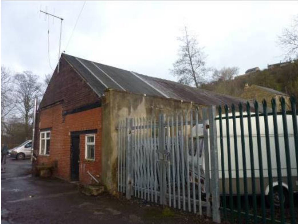
Photo 3: Building 1 viewed from the south
