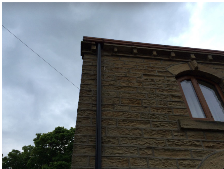
Photo 5: Close up of stonework (solid) & stone verge.
