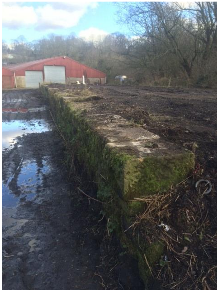
Reference Photographs; February 2016 Former Railway Station, Goods Yard Fold Farm Netherton
