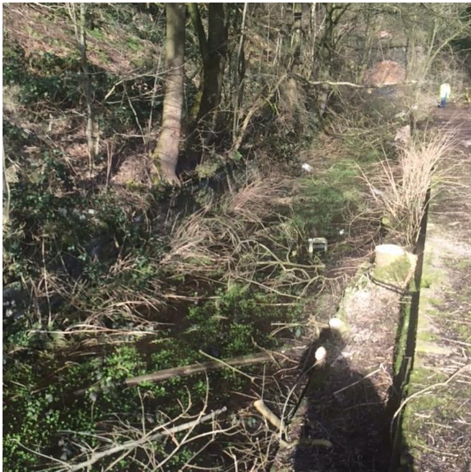
Reference Photographs; February 2016 Former Railway Station, Goods Yard Fold Farm Netherton
