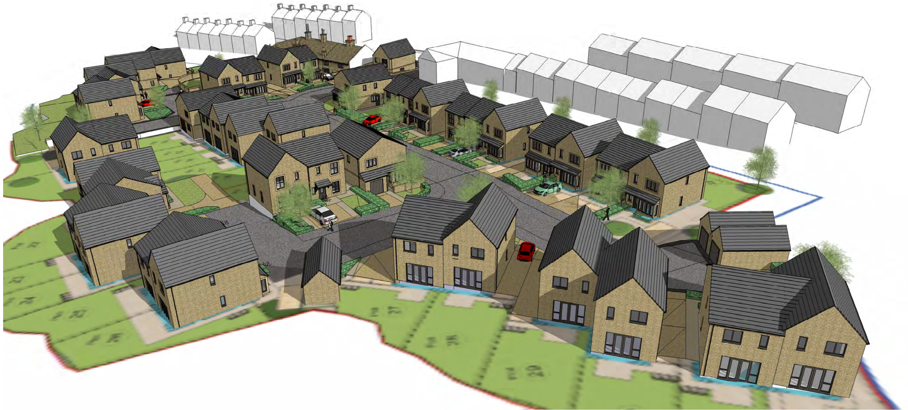
View A2 – Aerial view looking East
