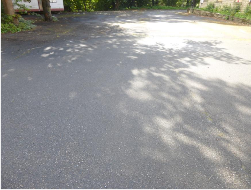
Photograph 11 – Car parking facilities are evident within the northern section of the site which consists of tarmacadam surfacing throughout. There were no signs of hydrocarbon contamination at the surface.
