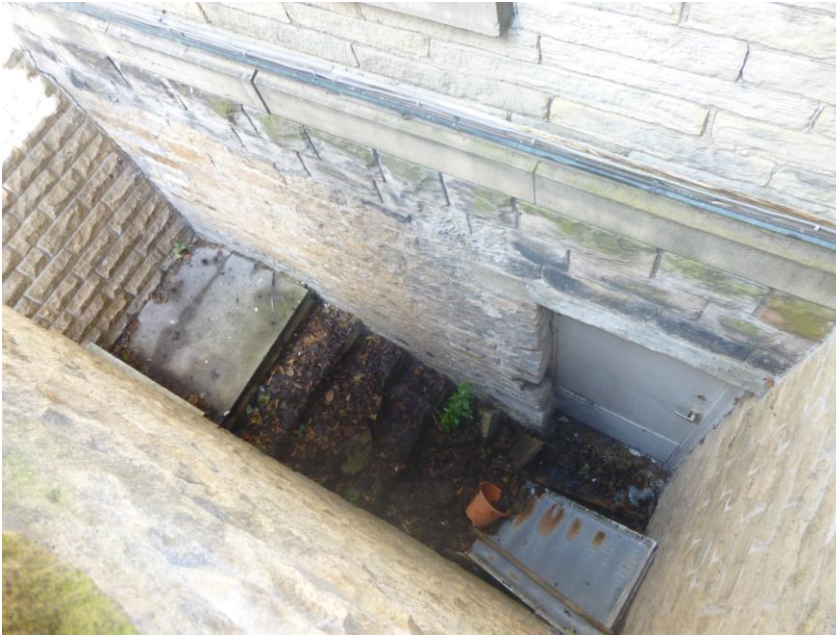
Photograph 17 – Showing the external staircase leading to a cellar.
