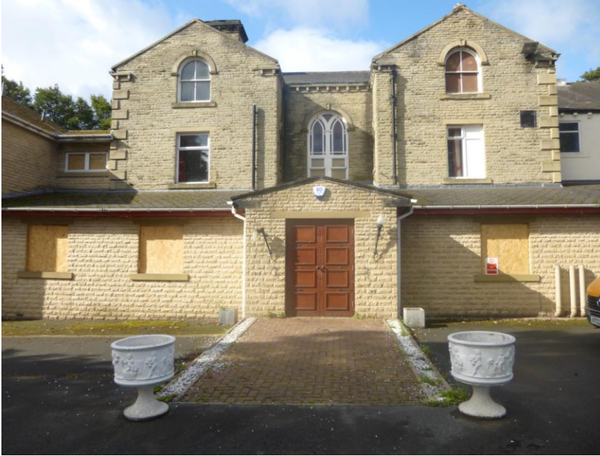
Photograph 9 – Showing the front elevation of the Hotel. The block paved ramp will have been used as an access point to the Hotel for residents.
