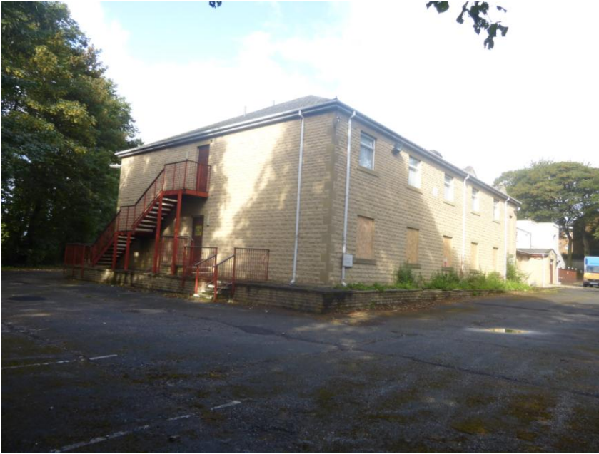
Photograph 13 – Showing the front elevation of the Hotel, looking in a south western direction.
