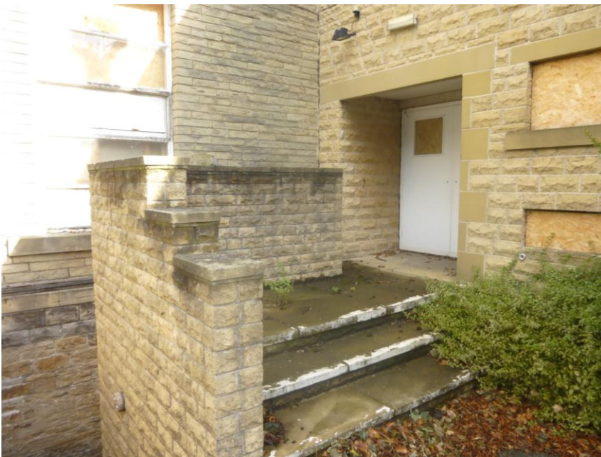
Photograph 16 – At the rear elevation of the property is a staircase leading to a cellar.
