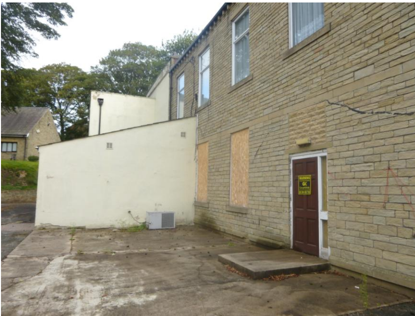
Photograph 20 – Showing the rear elevation of the Hotel, looking in a western direction.
