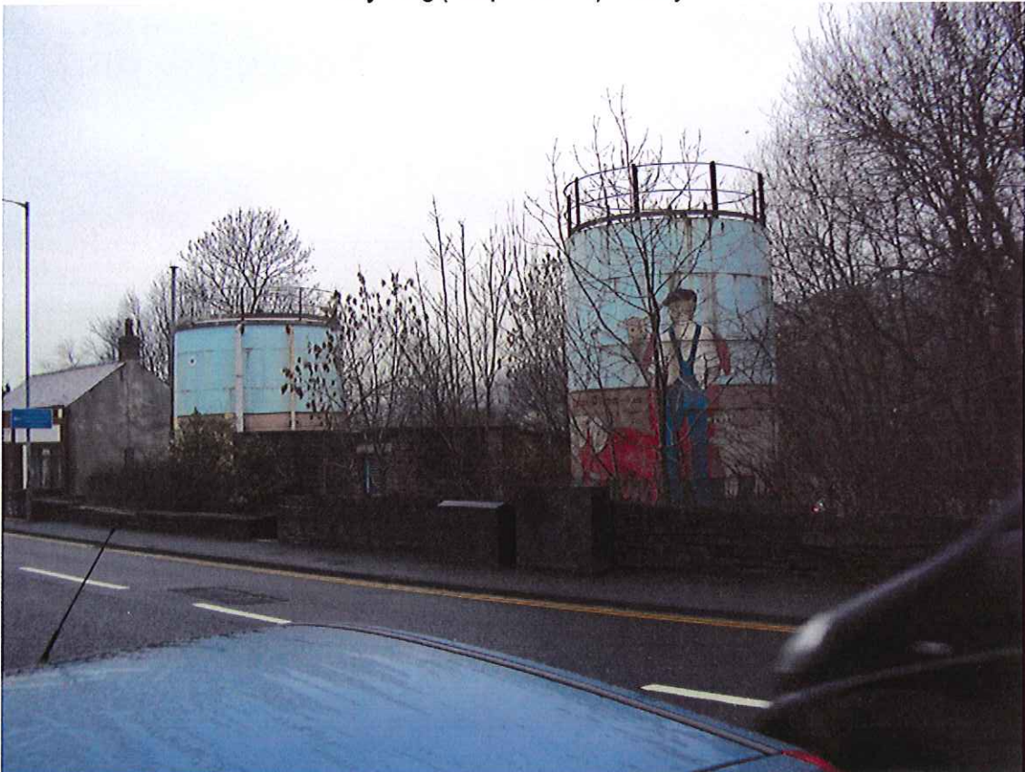
Photo – 4 View of site to the north west (Existing water treatment and effluent plant)
