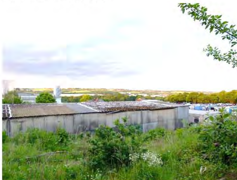
Plate 3. Buildings are of portal frame or block construction and offer negligible potential for use by bats
