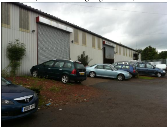
Photo 4. (View of MOT garages to NW)
